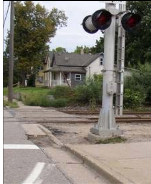
This railroad crossing on Marshall Avenue NE is an example of a location with complete sidewalks approaching the tracks, but an incomplete walking surface crossing the tracks.
