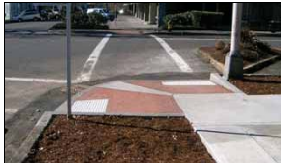
This curb ramp is an example of a design which could make it easier to fit two perpendicular curb ramps per corner than the current standard. Source: Accessible Public Rights of Way: Planning and Designing for Alterations , Institute of Transportation Engineers, July 2007.
