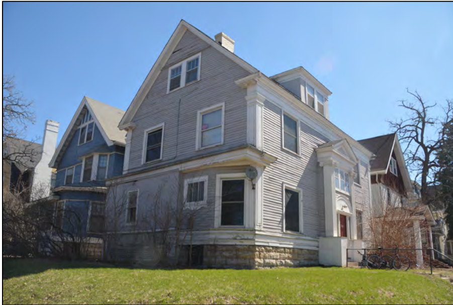
Fig. 5. West and north elevations of 1103 4th Street S.E.
