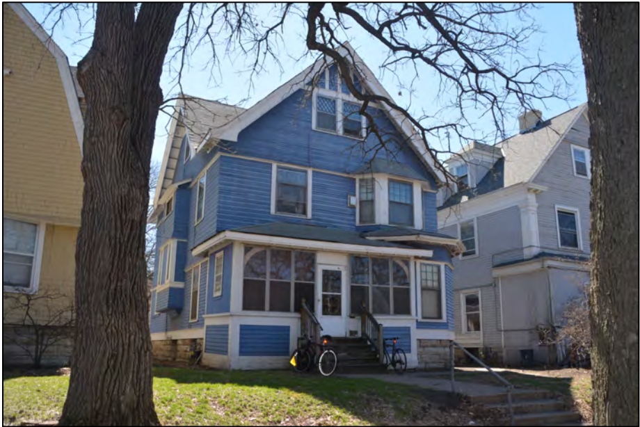
Fig. 8. West elevation of 406 11th Avenue S.E.
