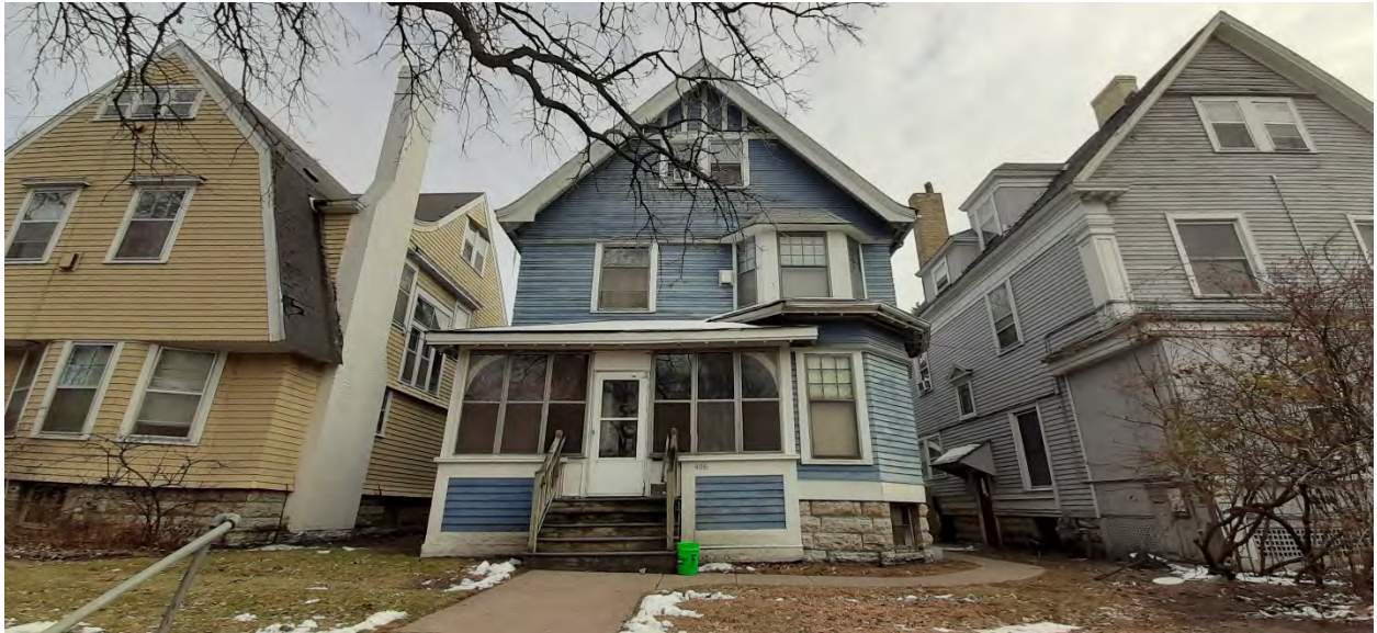
Front (west/northwest) elevation of 406 11 th Avenue SE, From 11 th Avenue SE, looking east/Southeast, November 2020, SOURCE: CPED
