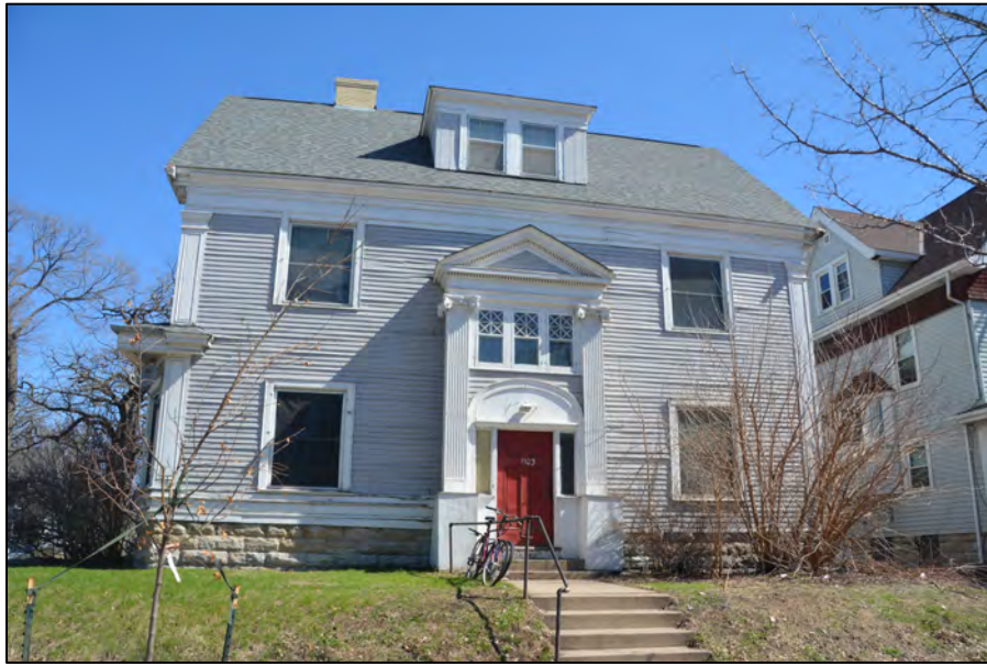
Figs. 4. West elevation of 1103 4th Street S.E.
