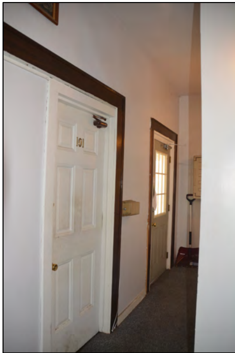
Fig. 12. First floor entrance, 410 11th Avenue S.E.
