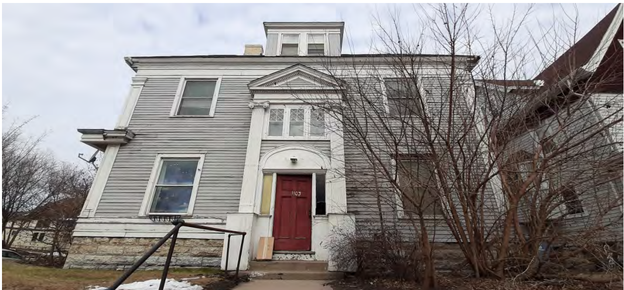
FIGURE 16. FRONT (SOUTH/SOUTHWEST) ELEVATION OF 1103 4 TH STREET SE, FROM 4 TH STREET SE, LOOKING NORTH/NORTHEAST, NOVEMBER 2020, SOURCE: CPED
