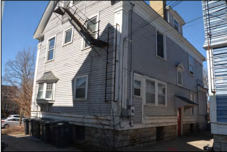
Fig. 6. East and south elevations of 1103 4th Street S.E.
