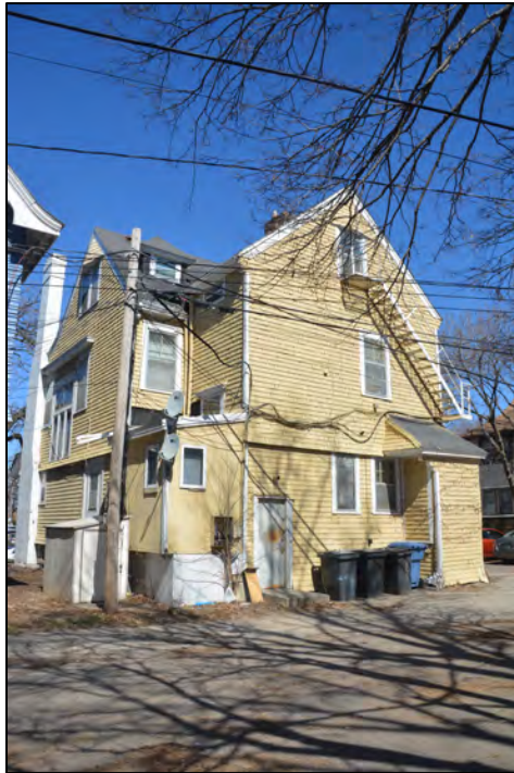
Fig. 11. West elevation of 410 11th Avenue S.E.
