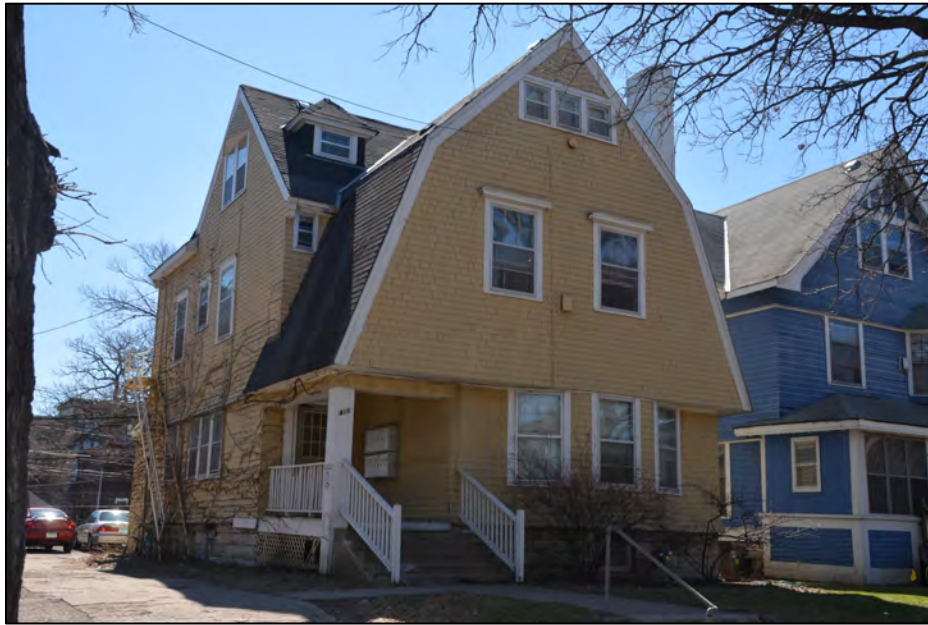
Fig. 10. East Elevation of 410 11th Avenue S.E.
