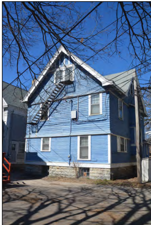
Fig. 9. East elevation of 406 11th Avenue S.E.
