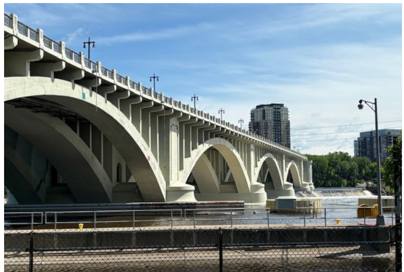
View of the recently restored 3rd Avenue bridge over the Mississippi River in Minneapolis. City water crews rehabilitated the water main that runs under the bridge deck as part of this project.
