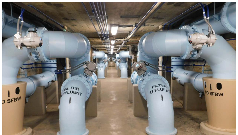
View of newly renovated pipe gallery at Minneapolis' Fridley Filter Plant.
