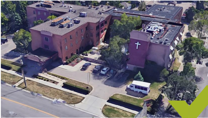
31 st and Lyndale Ave S Redeemer Residence, 105,000 sqft
