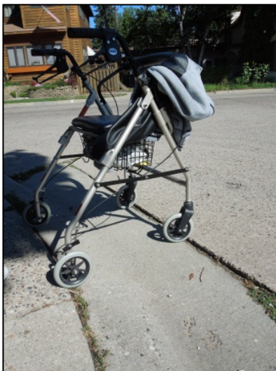
18th Ave NE & NE Polk St: A gutter pan sunk below street level catches the wheels on a resident's walker
