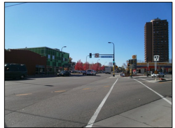
E Franklin Ave & Riverside Ave: Traffic signal with green arrow for right turns is confusing for crossing pedestrians; the wide intersection is also intimidating.
