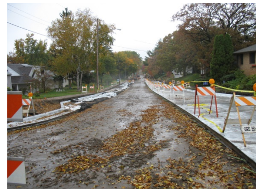
Example of construction staging on 54 th Street West
