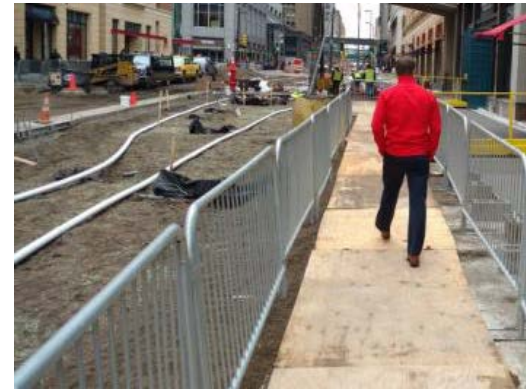
Example of temporary pedestrian access on downtown street
