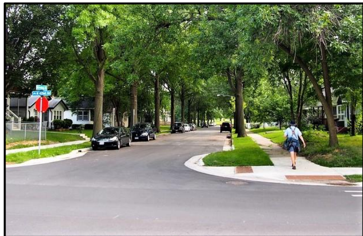
Figure F-6. Permanent Curb Extensions
