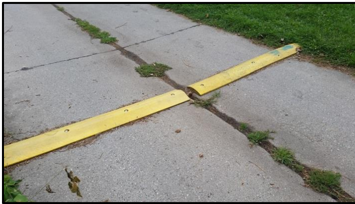
Figure F-22. Alley Speed Bump
