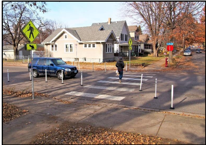
Figure F-5. Temporary Curb Extensions
