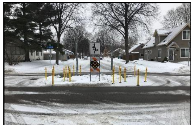
Figure F-10. Temporary Traffic Circle in Winter
