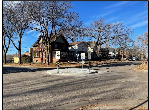
Figure F-9. Concrete Traffic Circle
