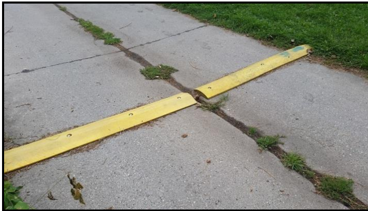
Figure F-22. Alley Speed Bump
