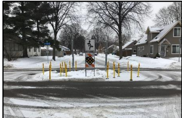
Figure F-10. Temporary Traffic Circle in Winter
