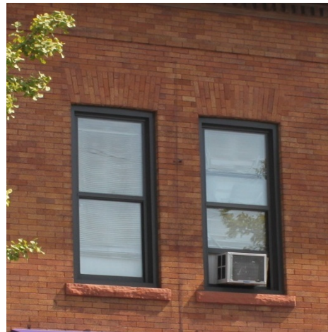
Flat brick arch over window
