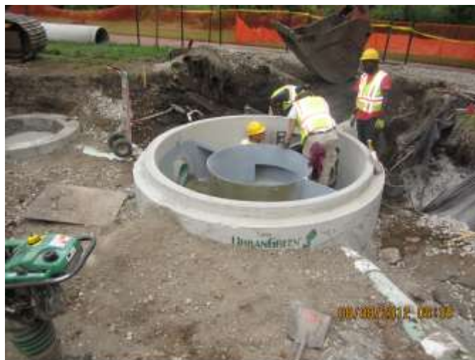
Grit Chamber Construction at Dean Pkwy
