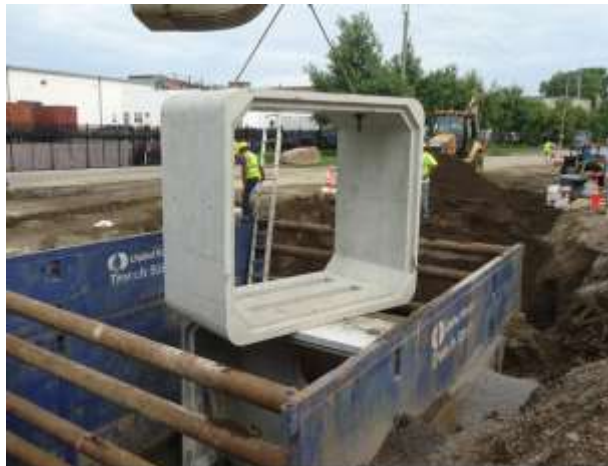
12x10 Infiltration Box Culvert Installation
