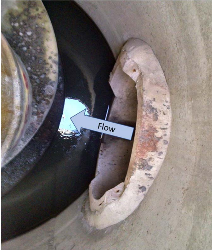
Figure 14-10. Photograph of the 36 inch south inlet at 24 th & Elm prior to equipment installation. Note the hydrodynamic separator downstream on the left. The blue arrow shows the direction of flow.
