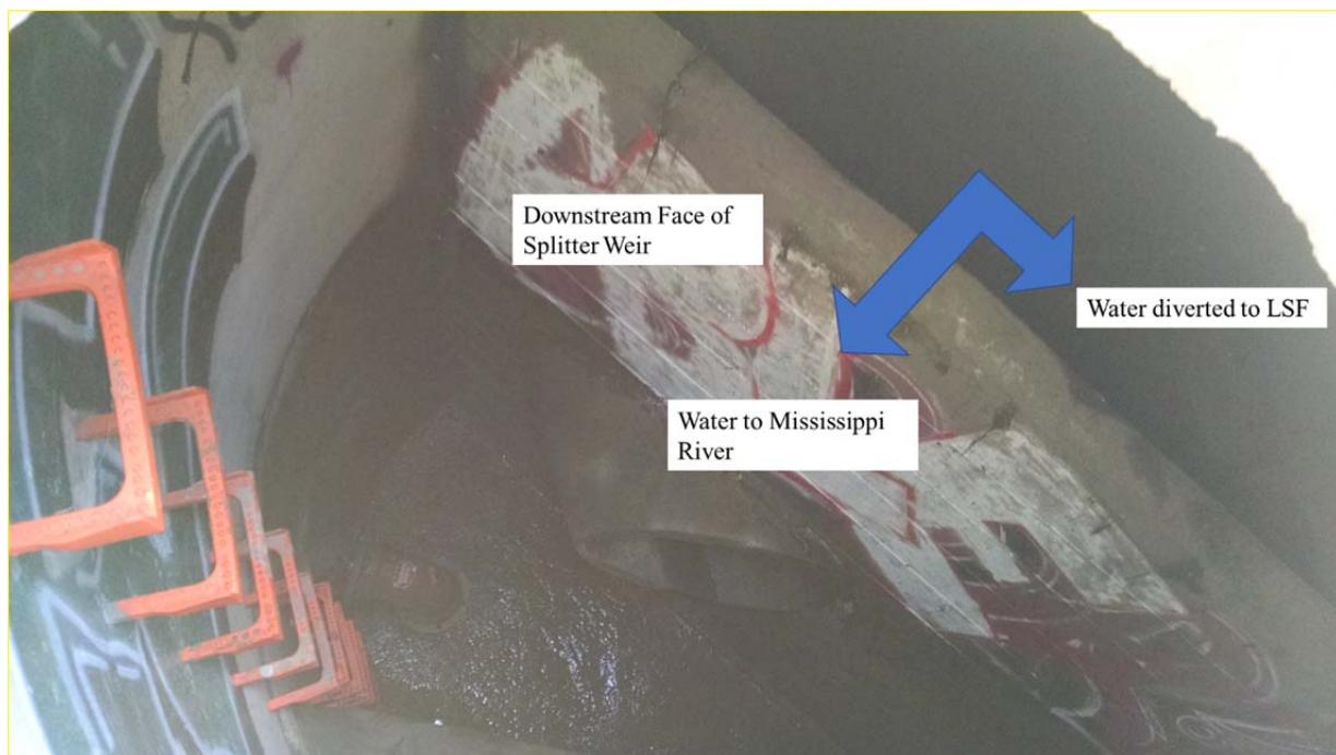
Figure 14-3. Downstream Photo of the flow splitter weir to the Lowry Sand Filter.
