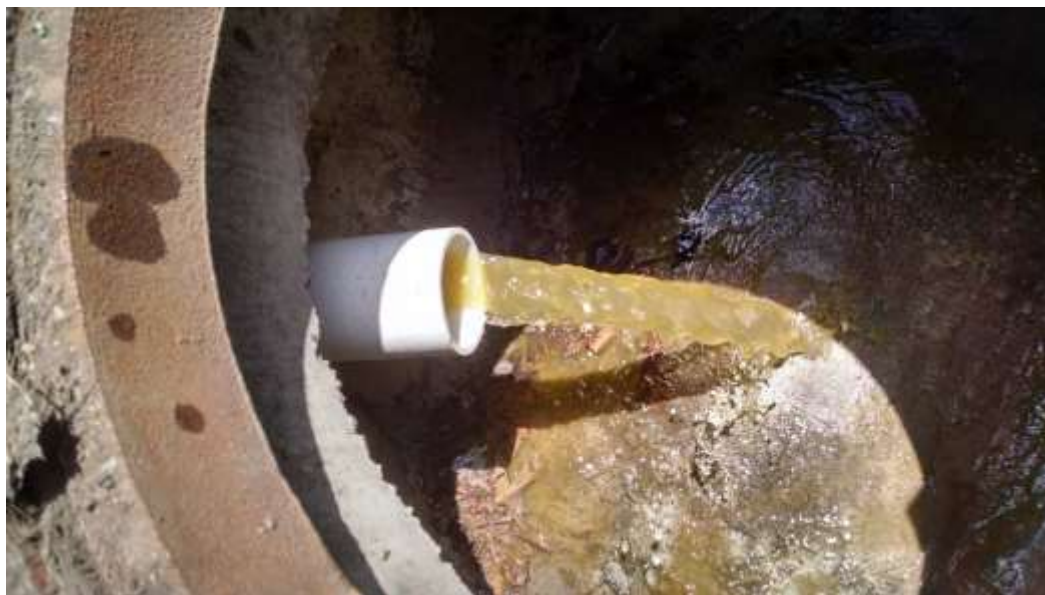
Figure 14-36. The washing machine discharges to the storm sewer.
