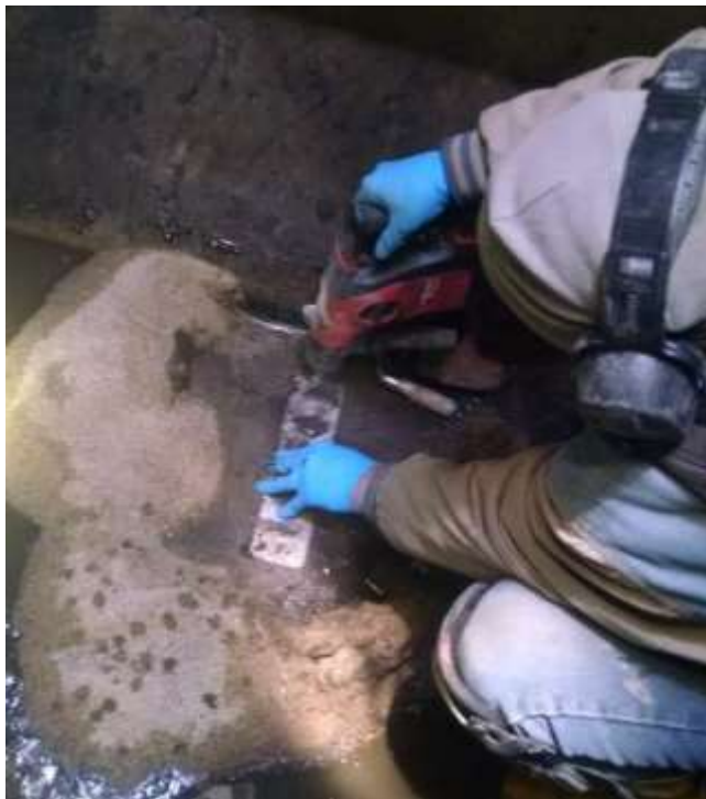
Figure 14-23. AV Anchor plate being installed in the vault floor.
