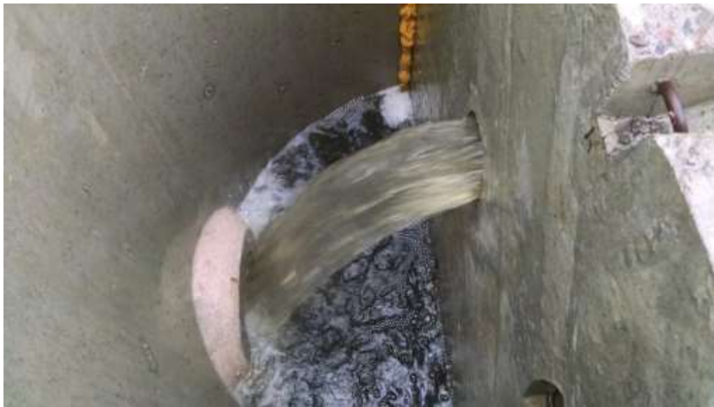
Figure 14-33. Webber Pond Outlet orifice discharging water into the 12 inch RCP Outlet. At the top of picture note the leaky orange expandable foam sealing the downstream weir side joint.
