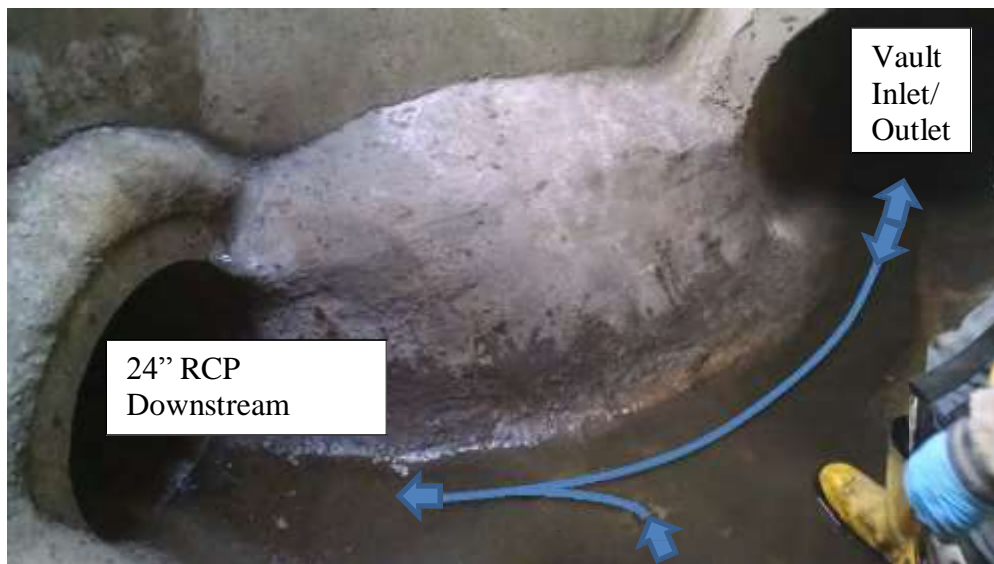
Figure 14-24. The vault entrance/exit pipe (right) and 24" downstream pipe (left).
