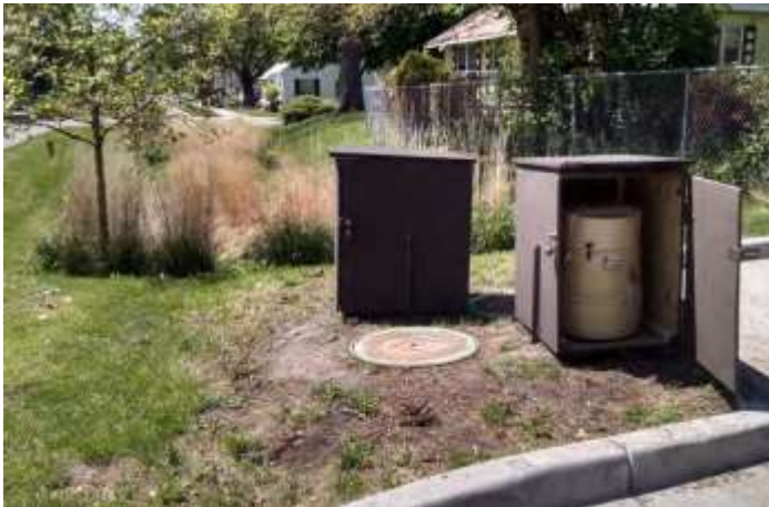
Figure 14-9. The 37 th Alley Site. Each enclosure contains a sampler, one for the Inlet and one for the Outlet.
