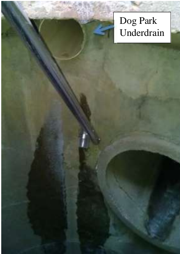
Figure 14-42. View inside the manhole of Lyndale Farmstead Dog Park. The small 6" PVC pipe at the top is the Lyndale Dog Park outlet.
