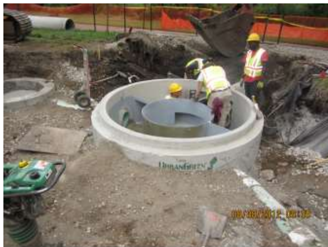
Grit Chamber Construction at Dean Pkwy
