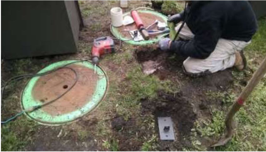
Figure 14-8. Mounting sub-surface anchor brackets for the sampler enclosure structures.
