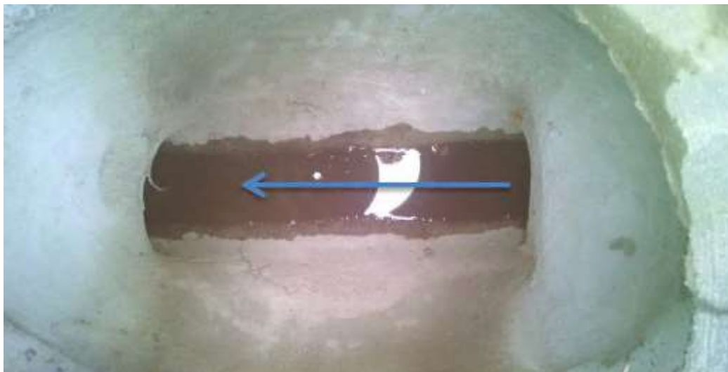
Figure 14-34. Webber Outlet 12-inch RCP pipe. Arrow shows direction of flow towards Shingle Creek.
