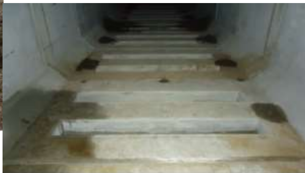
Infiltration Box Culvert – inside view
