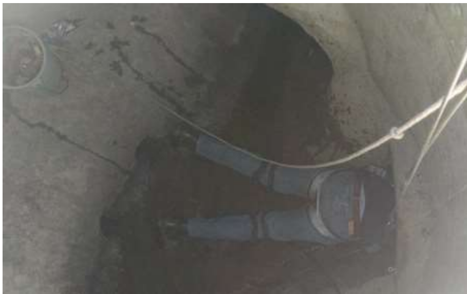
Figure 14-25. Installation of the spring ring in the 24" downstream pipe.
