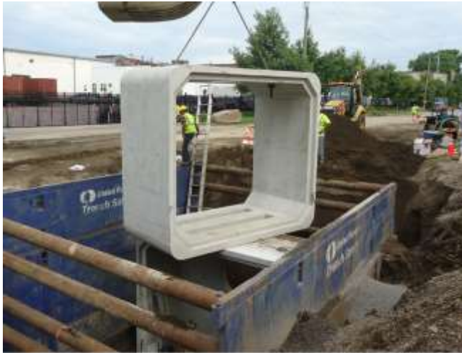
12x10 Infiltration Box Culvert Installation
