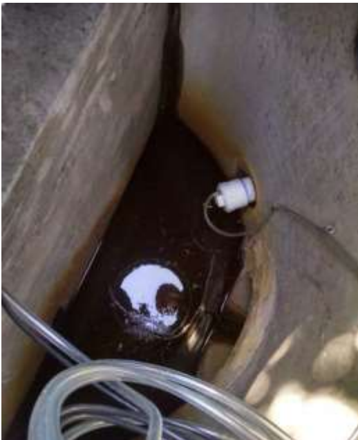
Figure 14-5. Photograph of the 4-inch (white) PVC outlet structure from the IESF. In 2016, the threaded end caps, present here, were removed to improve ventilation.
