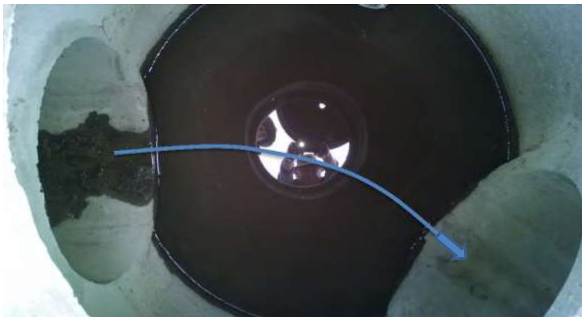
Figure 14-31. Webber South Inlet 24 inch RCP pipe. Arrow shows direction of flow. A sump is between the two pipes.
