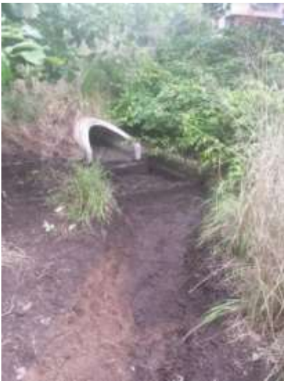
Figure 14-4. Flared end section and splash block inlet structure to the IESF.
