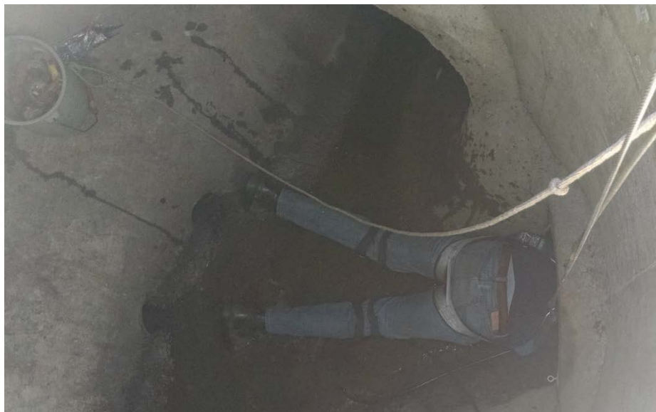
Figure 14-25. Installation of the spring ring in the 24" downstream outlet pipe.
