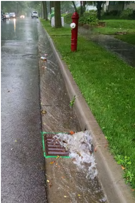
Figure 14-3 Stormwater flowing into a control catch basin at 37 th & Morgan.
