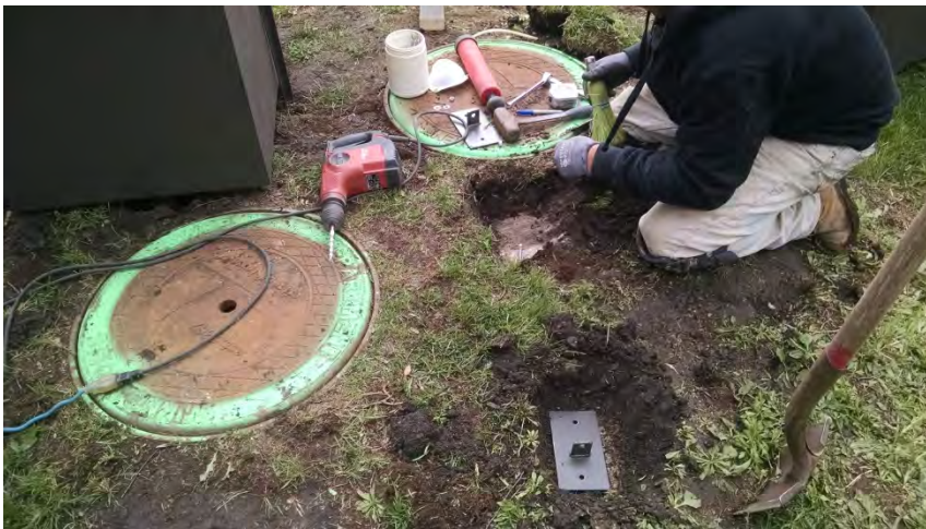
Figure 14-11. Mounting sub-surface custom anchor brackets for the sampler enclosure structures.
