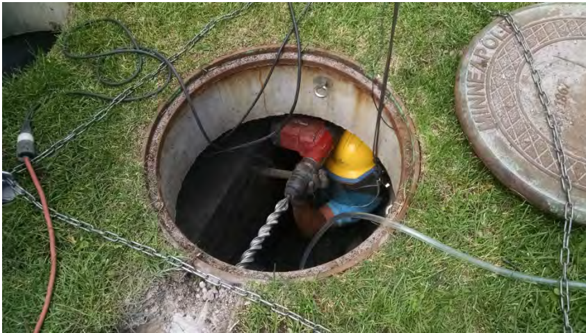
Figure 14-10. The cement shop drilling access holes and anchors.
