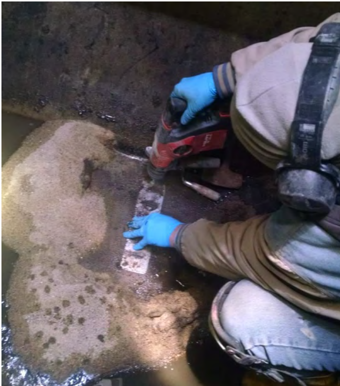
Figure 14-23. AV Anchor plate being installed in the vault floor.
