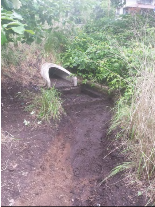
Figure 14-8: Flared End section and splash block inlet structure to the IESF.
