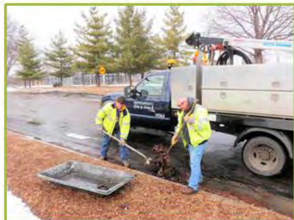
Cleaning debris from a plugged catch basin
