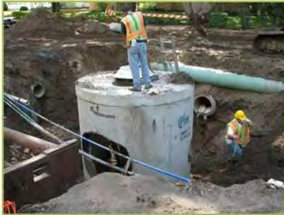
Hydrodynamic separator grit chamber being installed
