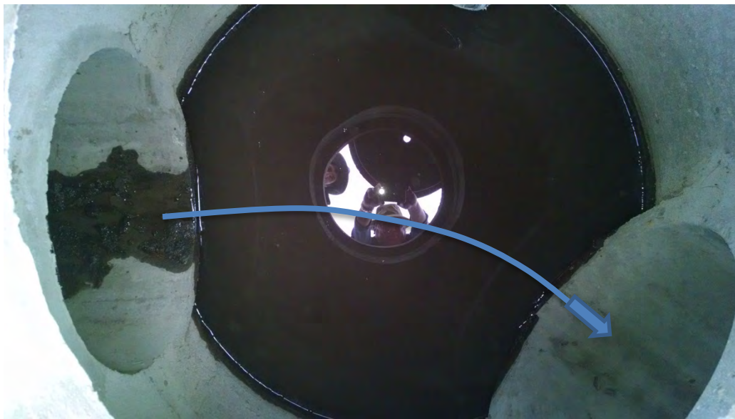
Figure 14-30. Webber South inlet 24 inch RCP pipe. Arrow shows direction of flow.
