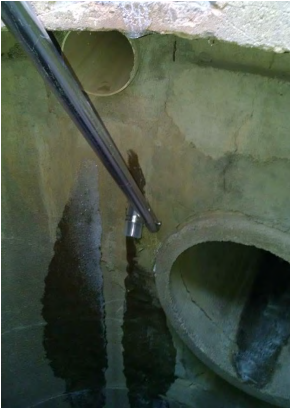
Figure 14-37. View inside the vault of Lyndale Farmstead Dog Park. The small PVC pipe at the top is the underdrain to the dog park.
