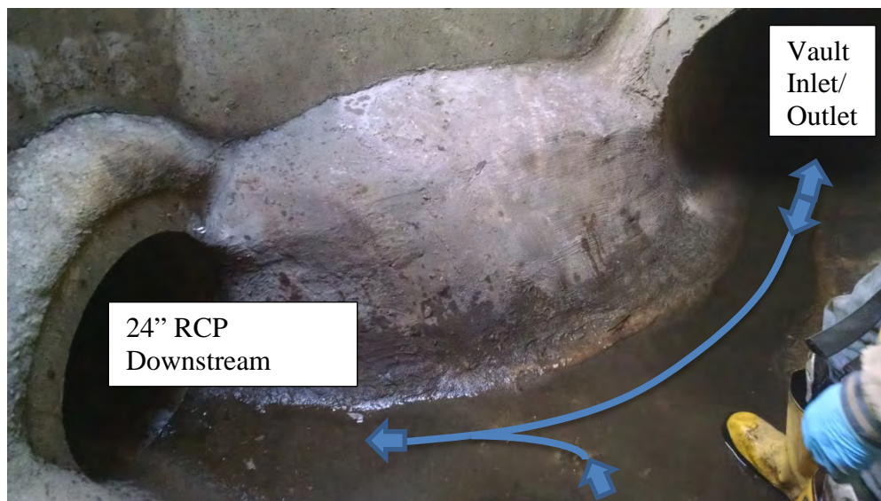
Figure 14-24. Photograph showing the vault entrance/exit pipe (right) and 24" downstream storm sewer outlet (left).
