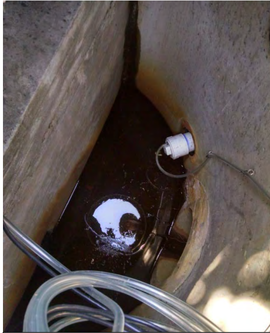
Figure 14-9: Photograph of the 4-inch (white) PVC outlet structure from the IESF.
