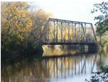
Boom Island Park Bridge
