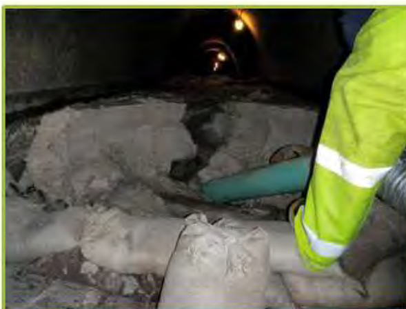
Removing sediment and eroded sandstone/limestone from 72" storm tunnel
