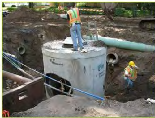
Hydrodynamic separator grit chamber being installed
