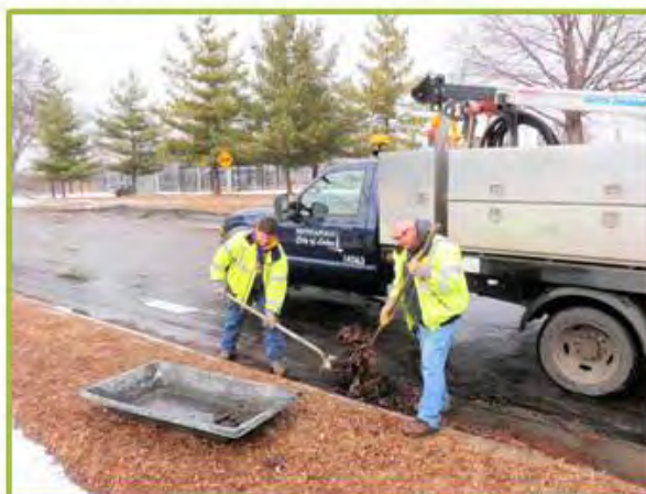
Cleaning debris from a plugged catch basin
