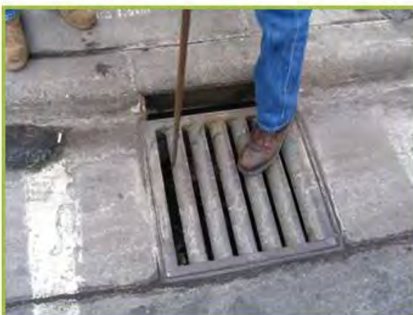
Photo of catch basin – an inlet to the storm drain system
