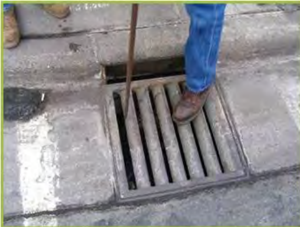
Photo of catch basin – an inlet to the storm drain system
