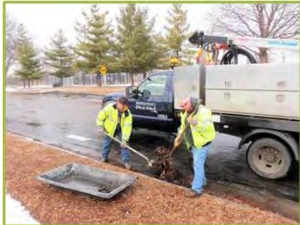
Cleaning debris from a plugged catch basin
