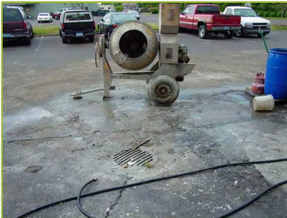
Construction site inspections also target concrete washout violations
