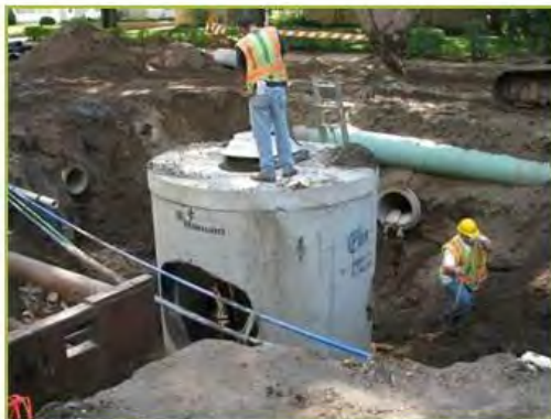
Hydrodynamic separator grit chamber being installed
