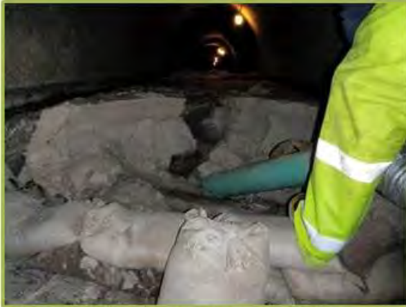
Removing sediment and eroded sandstone/limestone from 72" storm tunnel
