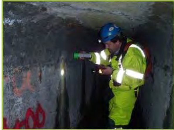
Inspecting a deep drainage tunnel, about 80 ft. underground
