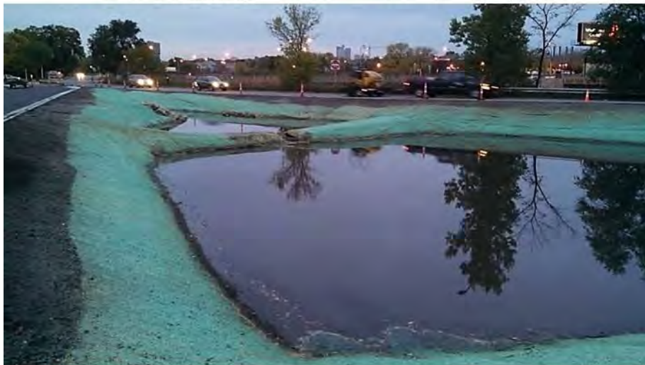
★ Winter Street 3-cell pond. 2013-2014 construction. Pond discharges to the I-35W (north) tunnel.
