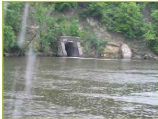
Large stormwater outfall to Mississippi River
