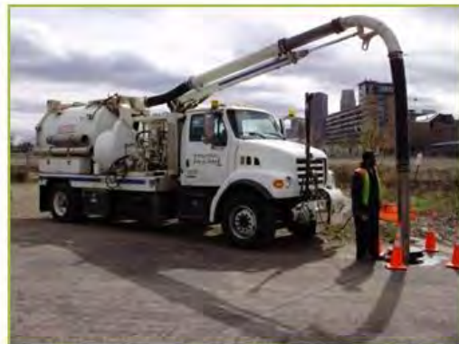
Grit chamber being vacuumed to remove sediments, oil and grease, trash and other debris
