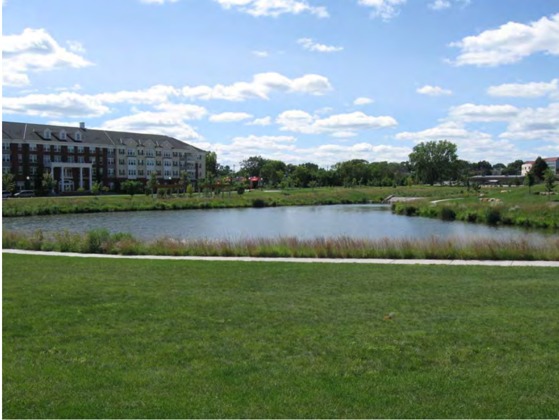
Figure 25-6. The Heritage Commons final pond looking west.
