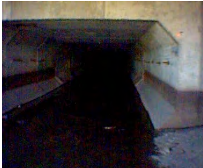
Figure 25-4. The Heritage Park Pond outlet following removal of the weir.
