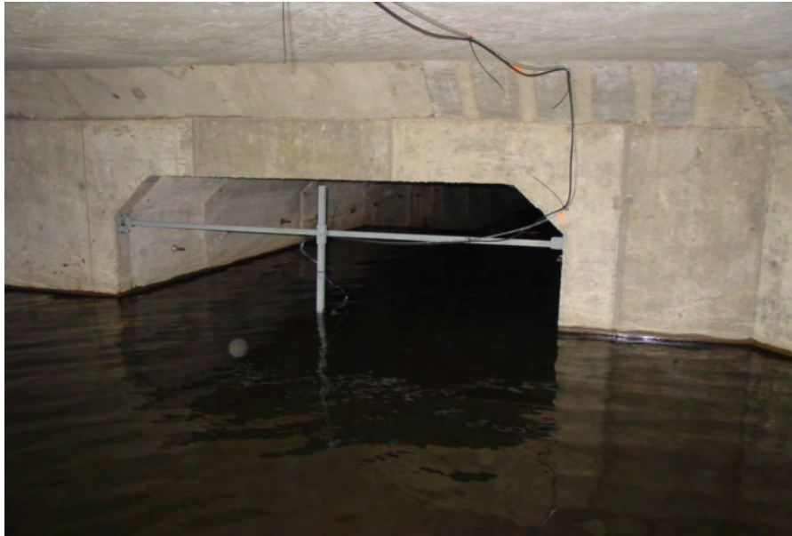
Figure 25-5. Heritage Park Pond box culvert with monitoring equipment installed.
