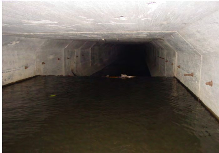
Figure 25-3. The Heritage Park Pond outlet weir is inside the 5' X 10' box culvert. Weir was removed on 9/3/08.
