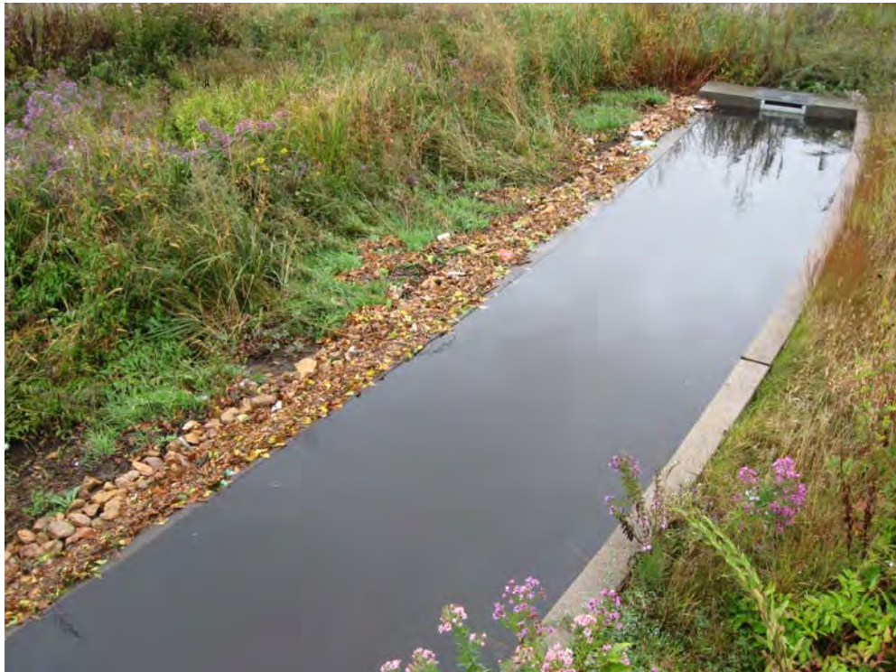
Figure 25-8. The Heritage Park infiltration basin 10/2/09 following 1.5 inch storm.
