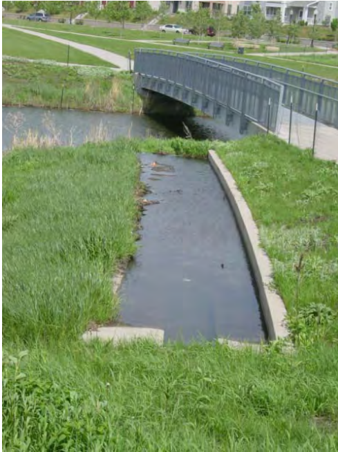
Figure 24F. Trench forebays not infiltrating (A), because they are silted in (B).
