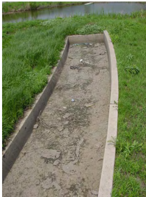
Figure 24F. Trench forebays not infiltrating (A), because they are silted in (B).
