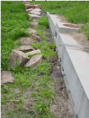
Figure 24G. Heritage Park with sediment in front of spreaders.
