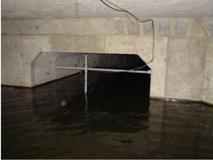
Figure 24D. Heritage Park Pond box culvert with monitoring equipment installed.
