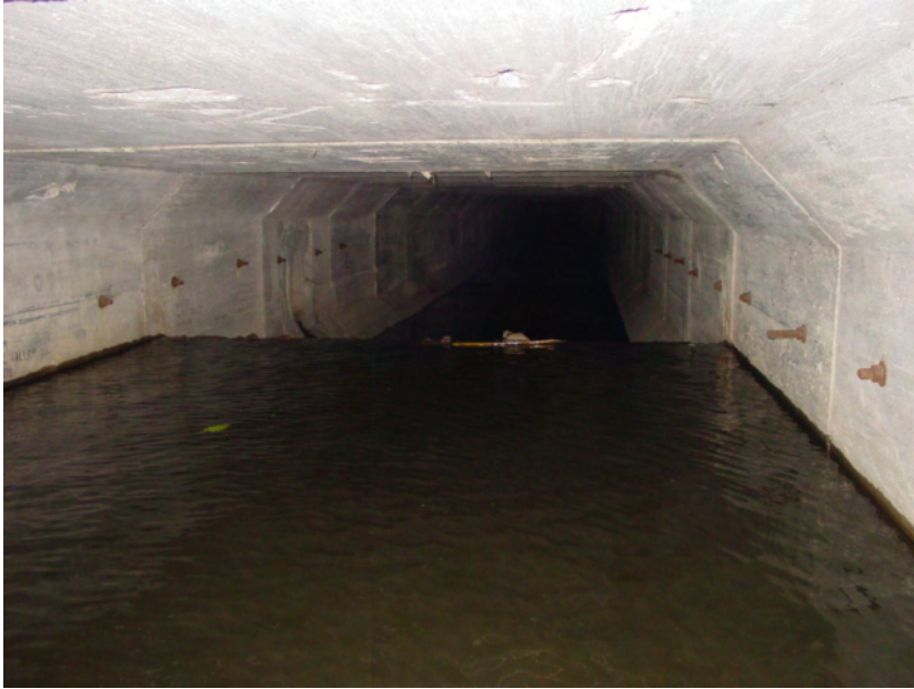
Figure 24C. The Heritage Park Pond weir is inside the 5' X 10' box culvert.
