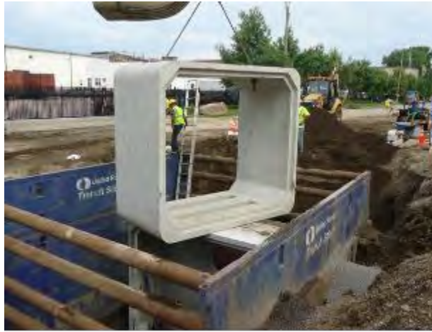
12x10 Infiltration Box Culvert Installation
