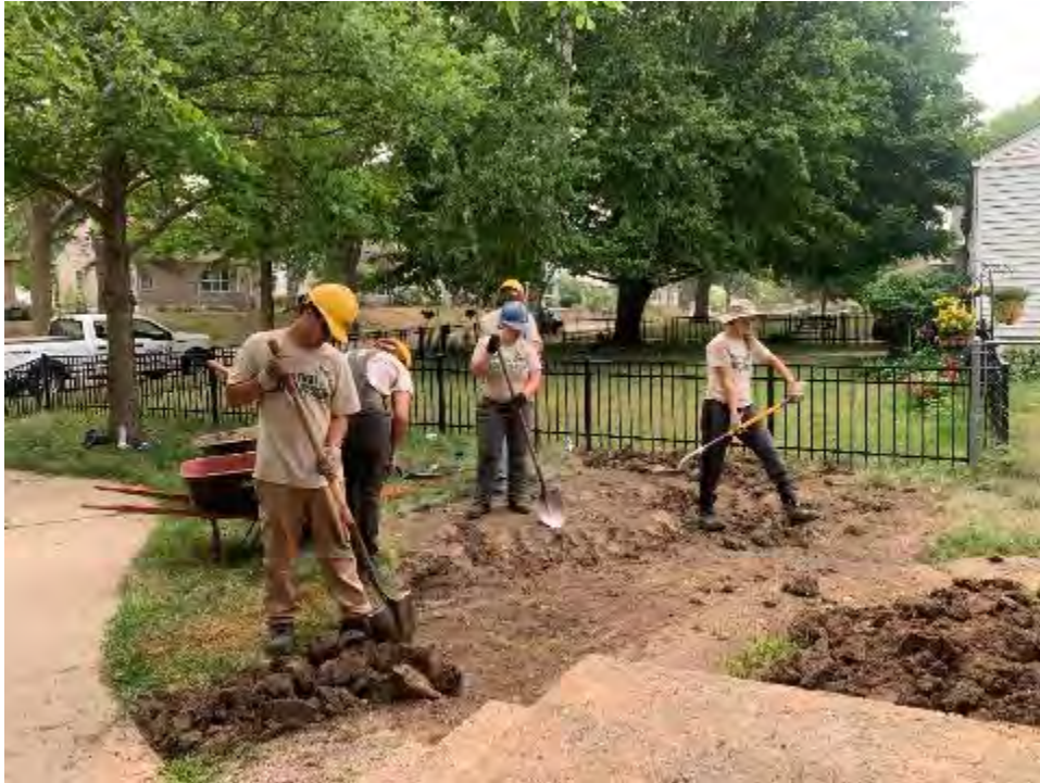
Figure 1-27 Conservation Corps crew working on one of the 100 raingardens installed
