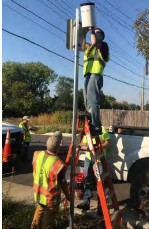
Figure 2. A rain gauge being installed at the Hoyer A GSI site in 2021.
