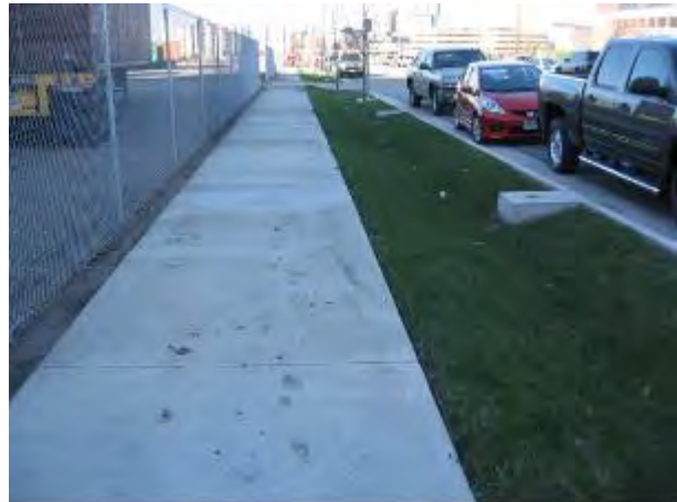
Vegetated Swale at 25 th Ave. SE
