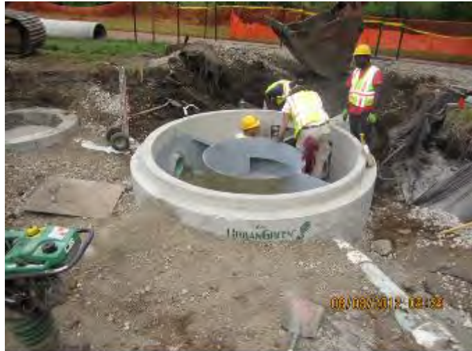
Grit Chamber Construction at Dean Pkwy
