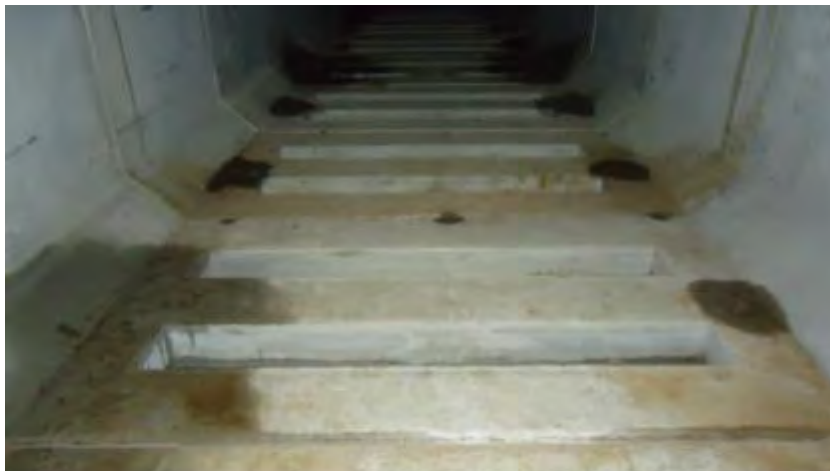
Infiltration Box Culvert – inside view
