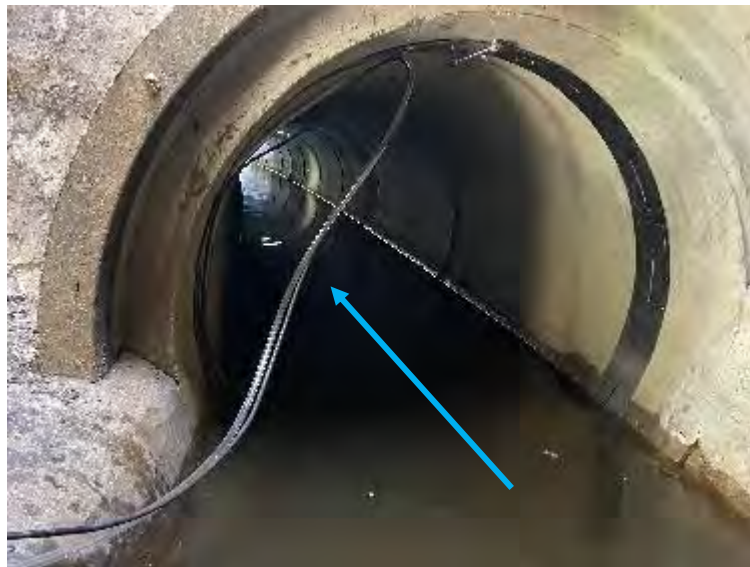
Figure 3. Photo of the spring ring at Camden Inlet S NW in May 2023. The blue arrow points in the direction of water flow.
