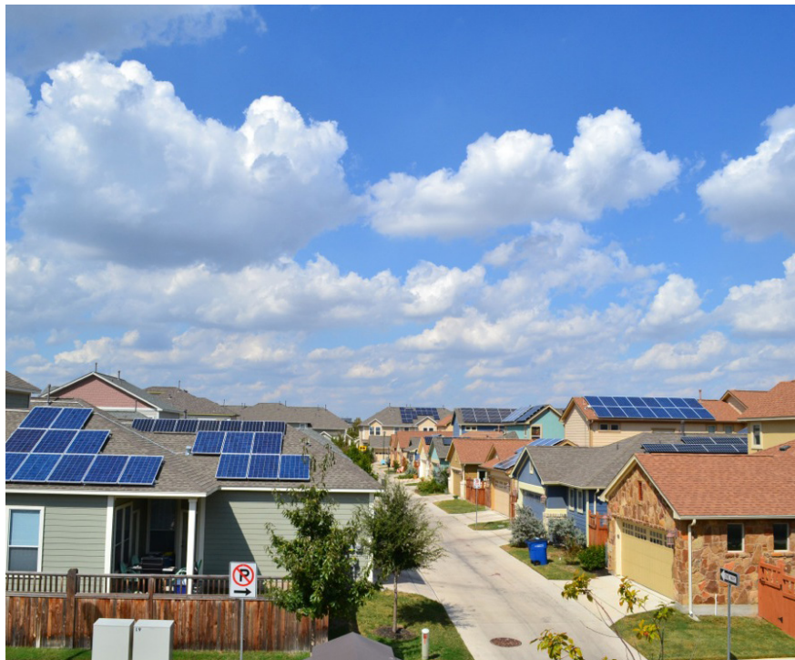
The Pecan Street Project homes.
