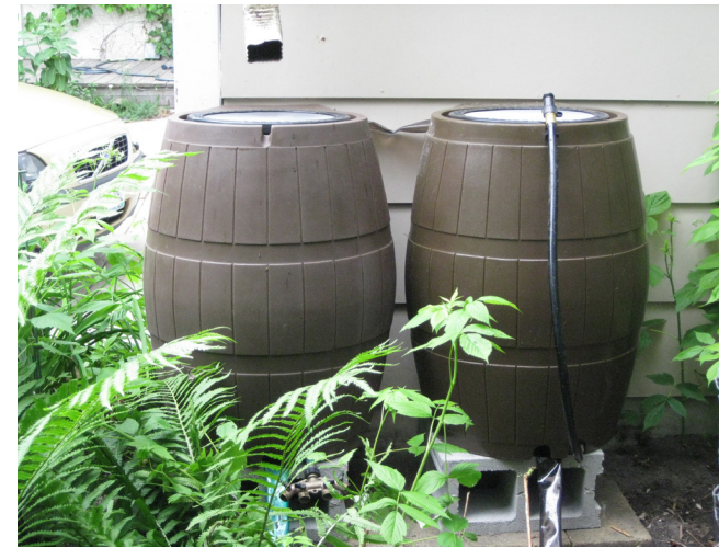
Two 60-gallon rain barrels installed in-series in Longfellow.
