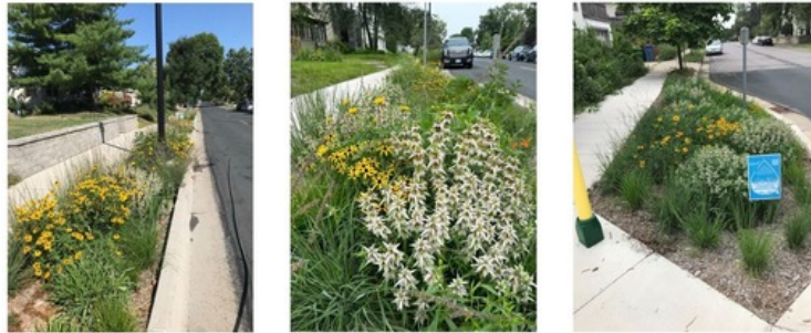
Completed rain garden basins
