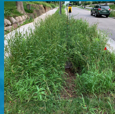
Unrestored rain garden basin, will be restored by City
