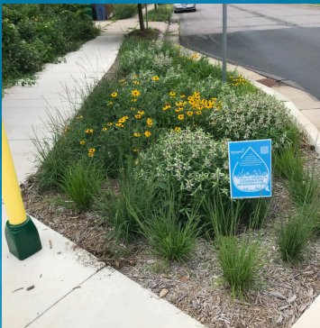
Restored rain garden basin
