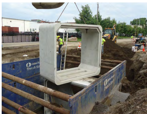
12x10 Infiltration Box Culvert Installation
