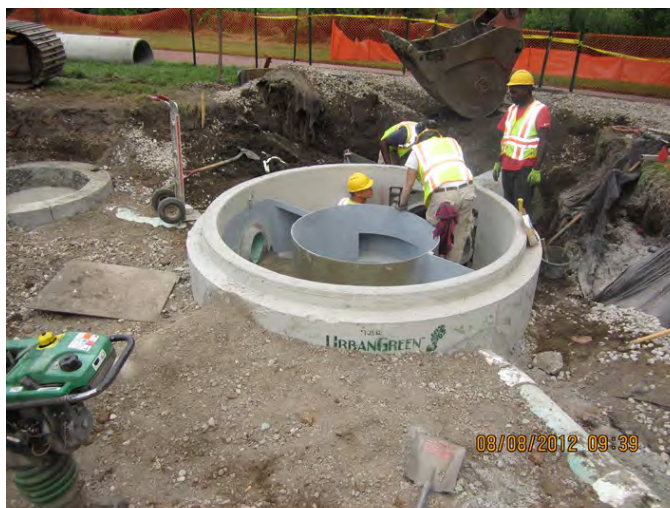
Grit Chamber Construction at Dean Pkwy
