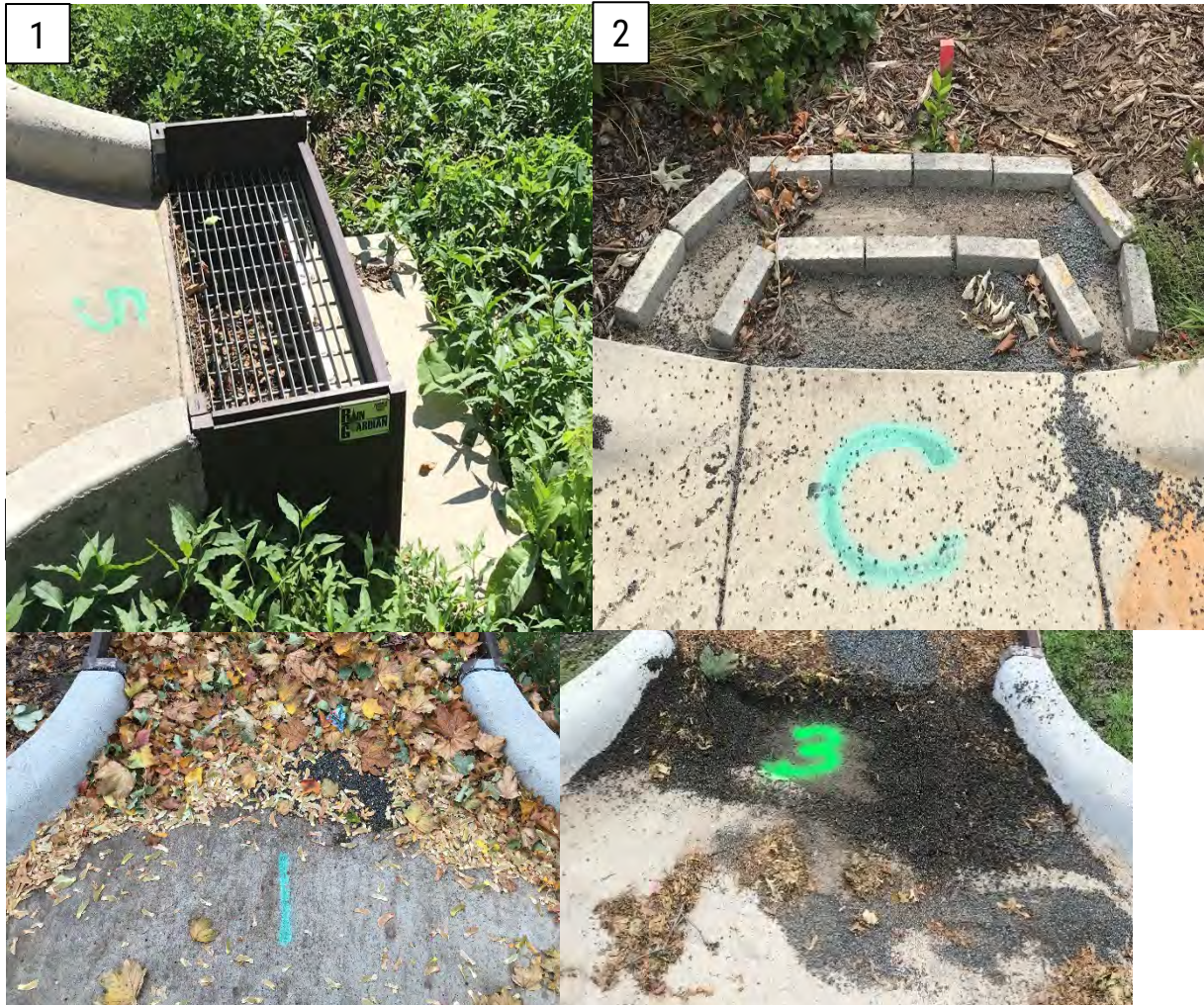
Figure 9. (1) A Windom pretreatment basin clogged with leaves in October 2022. (2) A Windom pretreatment basin clogged with sediment, soil, and leaves in June 2022.
