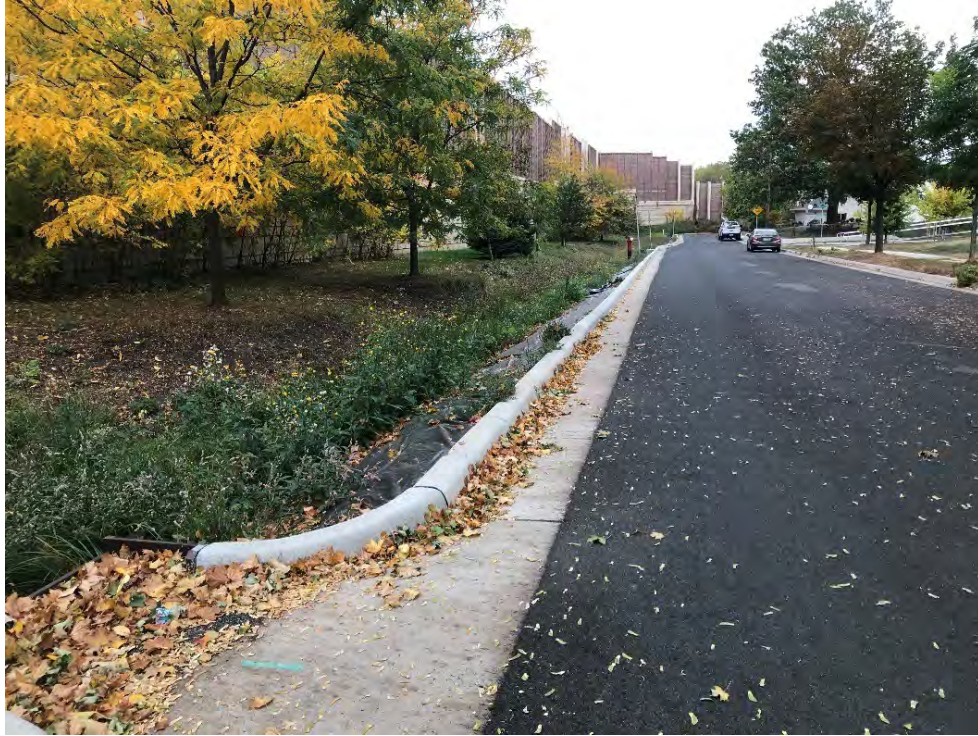
Figure 2. The Windom GSI basin in fall of 2022 in southwest Minneapolis. A Rain Guardian Bunker pretreatment basin filled with leaves can be seen in the lower left corner.
