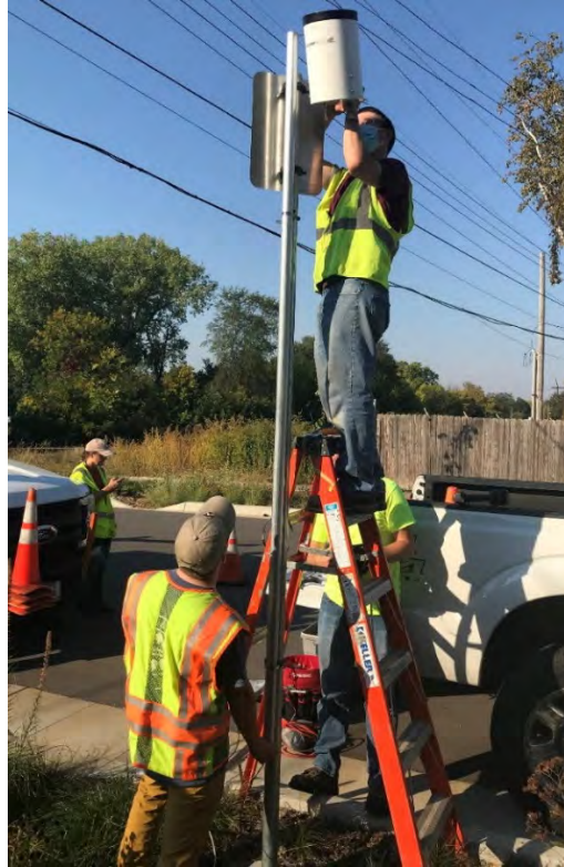
Figure 3. A rain gauge being installed at the Hoyer GSI site.
