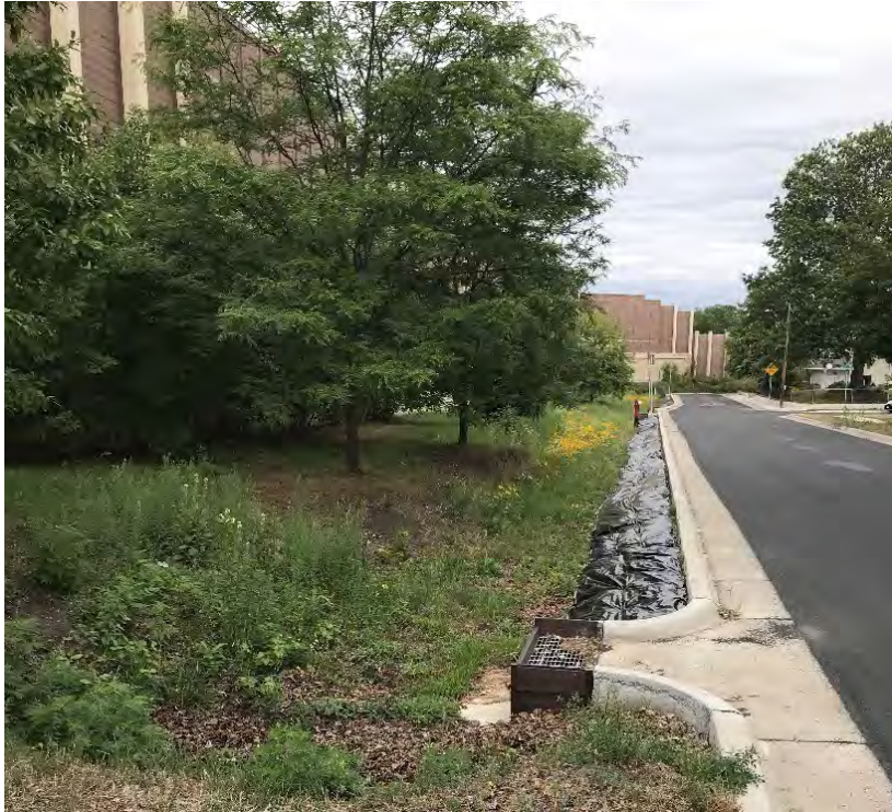
The Windom GSI site during the summer of 2022. One of five rain guardian bunker pretreatment systems are pictured.
