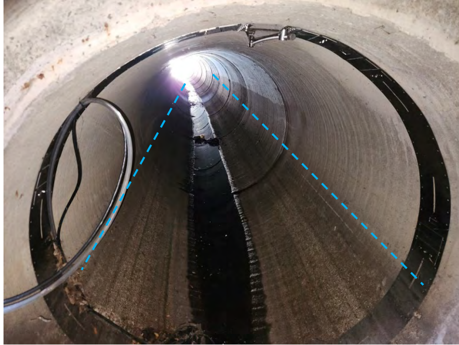
Figure 11. Image of Camden S NW pipe with some standing water. This image was taken at the end of the monitoring season, several months into a severe drought. Note the water line markings on the side of the pipe (blue dashed lines), showing the usual level of standing water.
