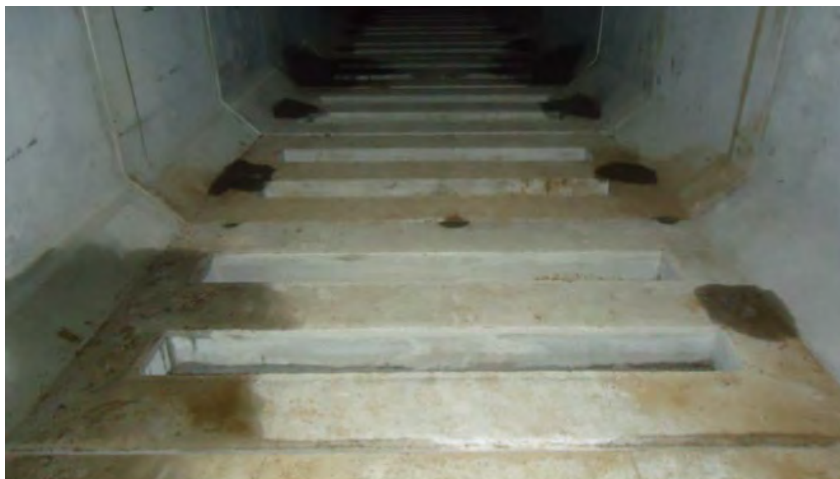
Infiltration Box Culvert – inside view
