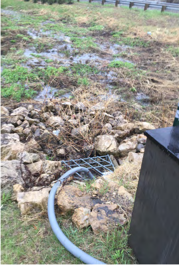
Figure 27-5. Photo of the WIB outlet. Standing water can be seen in the basin waiting to infiltrate and it has not reached the outlet. The brown box contains the monitoring equipment and the gray conduit armors the AV cable and sampler pump tubing.
