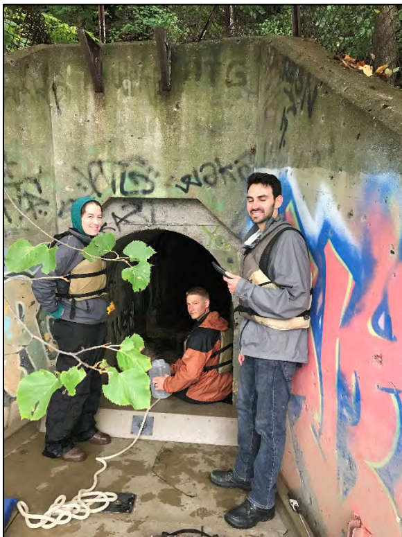
Minneapolis Public Works staff conducting a field dry weather flow screening
