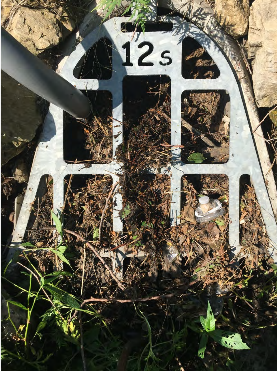
Figure 27-4. Photo of the west 12” inlet flared-end outfall and debris building up on the inside of the grate.
