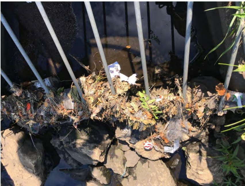
Figure 27-3. Looking upstream, a closer photo of the south inlet and trash building up on the inside of the grate.
