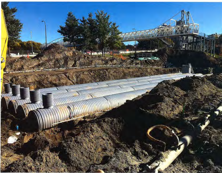
Figure 25-2. Photograph of the 80,000-gallon underground cistern under construction.
