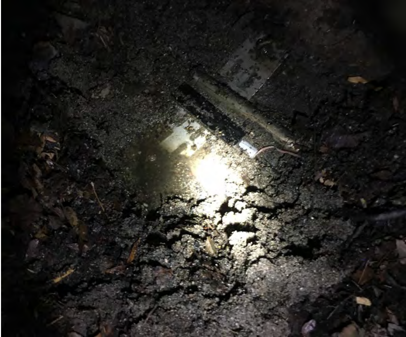
Figure 24-7. 2019 Powderhorn Inlet South offset AV probe and intake strainer after removing 8” of sand and debris.
