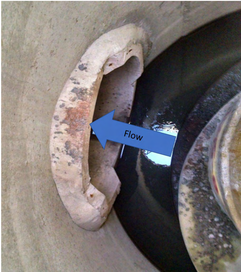
Figure 26-5. Photograph of the 36-inch north inlet at 24 th & Elm prior to equipment installation. Note the hydrodynamic separator upstream on the right. The blue arrow shows the direction of flow. Note, part of the pipe had to be cut away to allow access.
