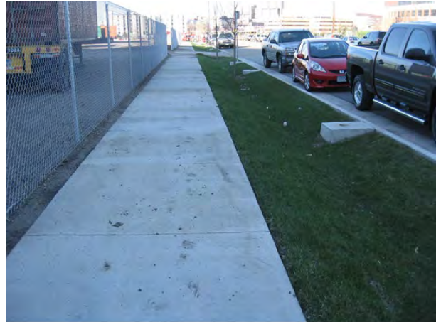
Vegetated Swale at 25 th Ave. SE
