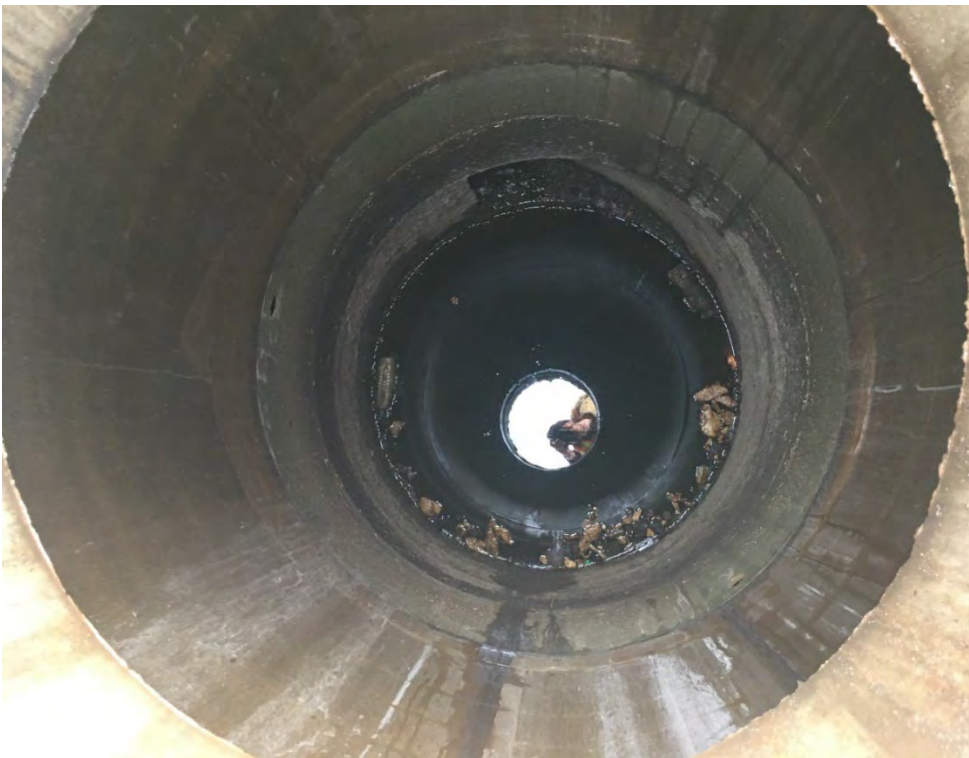
Figure 26-3. Photograph of the top clean-out manhole access of the north Contech hydrodynamic CDS separator.
