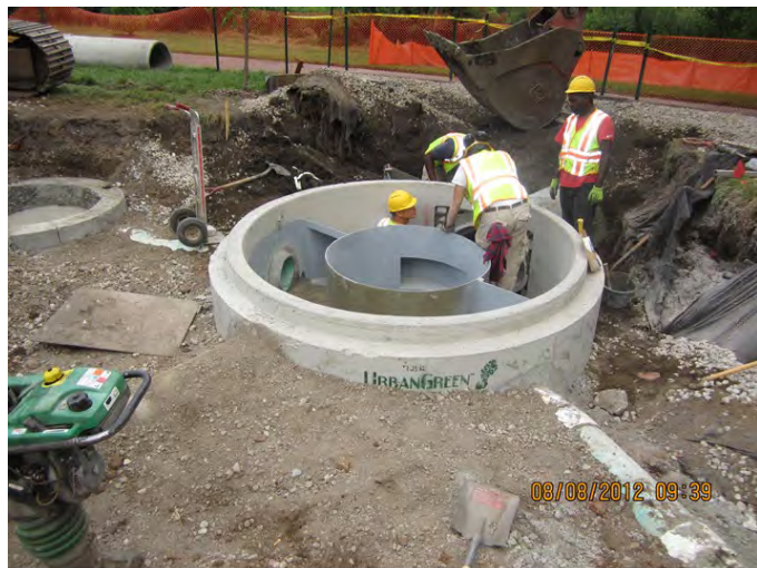
Grit Chamber Construction at Dean Pkwy
