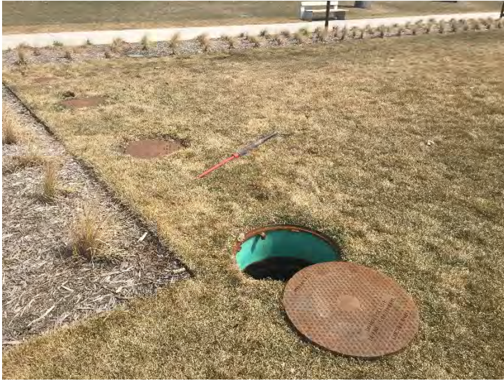
Figure 25-3. Photograph of the north manhole where sampling occurred at the underground cistern.
