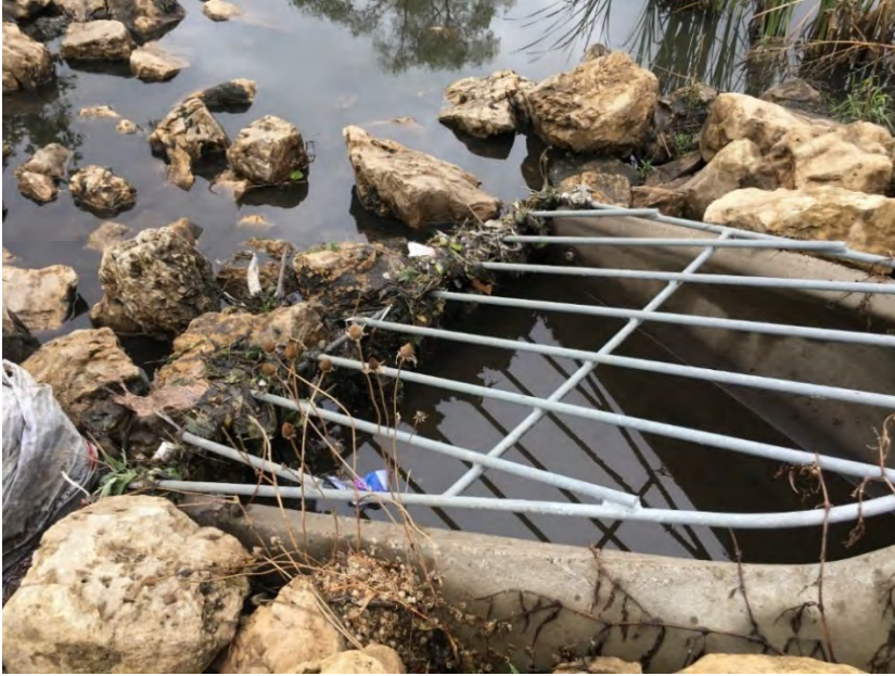
Figure 27-2. Photo of the south 24” inlet flared-end outfall and trash building up on the inside of the grate.
