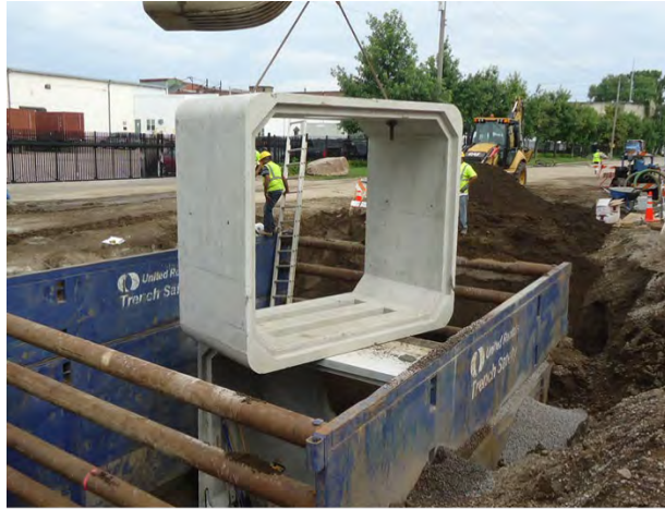
12x10 Infiltration Box Culvert Installation
