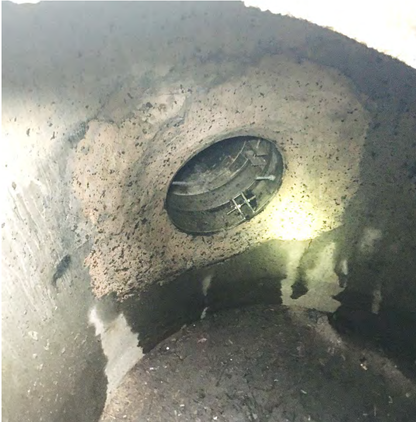
Figure 26-4. Photograph of the backflow preventer at 24 th Ave. SE, and Elm St. SE. The backflow preventer is approximately 36” above the 24 th pipe invert.
