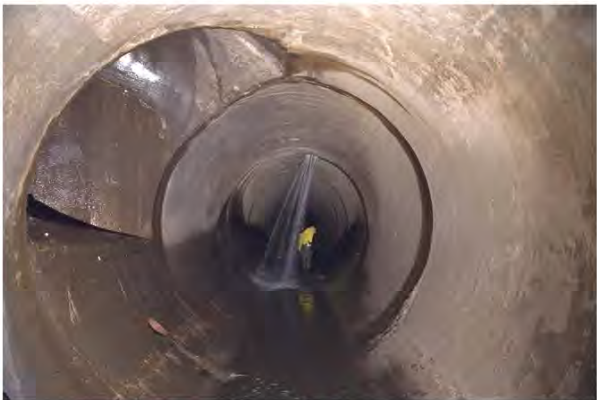
Water infiltrating into existing storm tunnel
