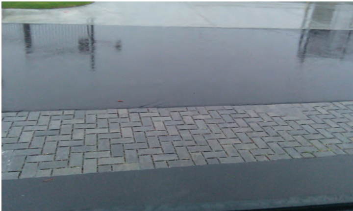
14th Ave NE - Infiltration with Pavers
