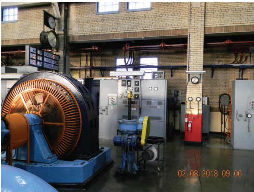
Motor Control Center (MCC) behind pump motor
