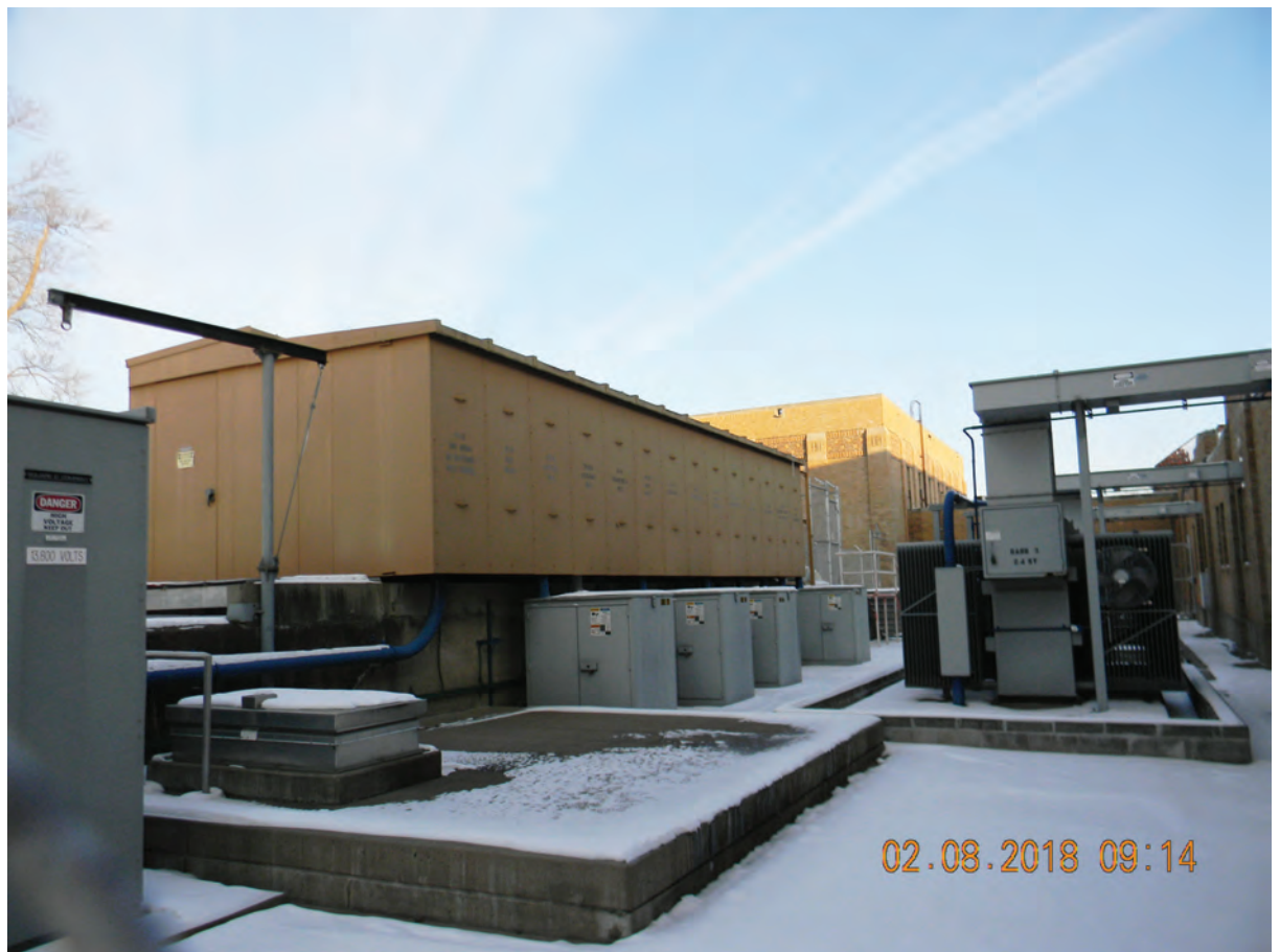
Incoming 13,800 volt switch house and transformers
