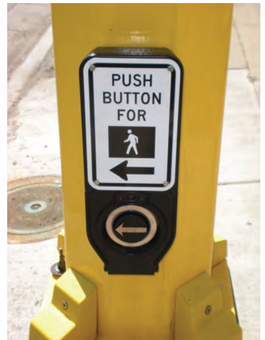
Accessible Pedestrian Signal
