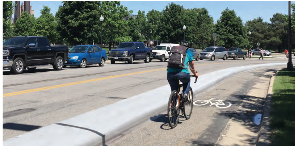
Illustrative rendering of curb protected bikeway - the City has installed this treatment on Oak St.
