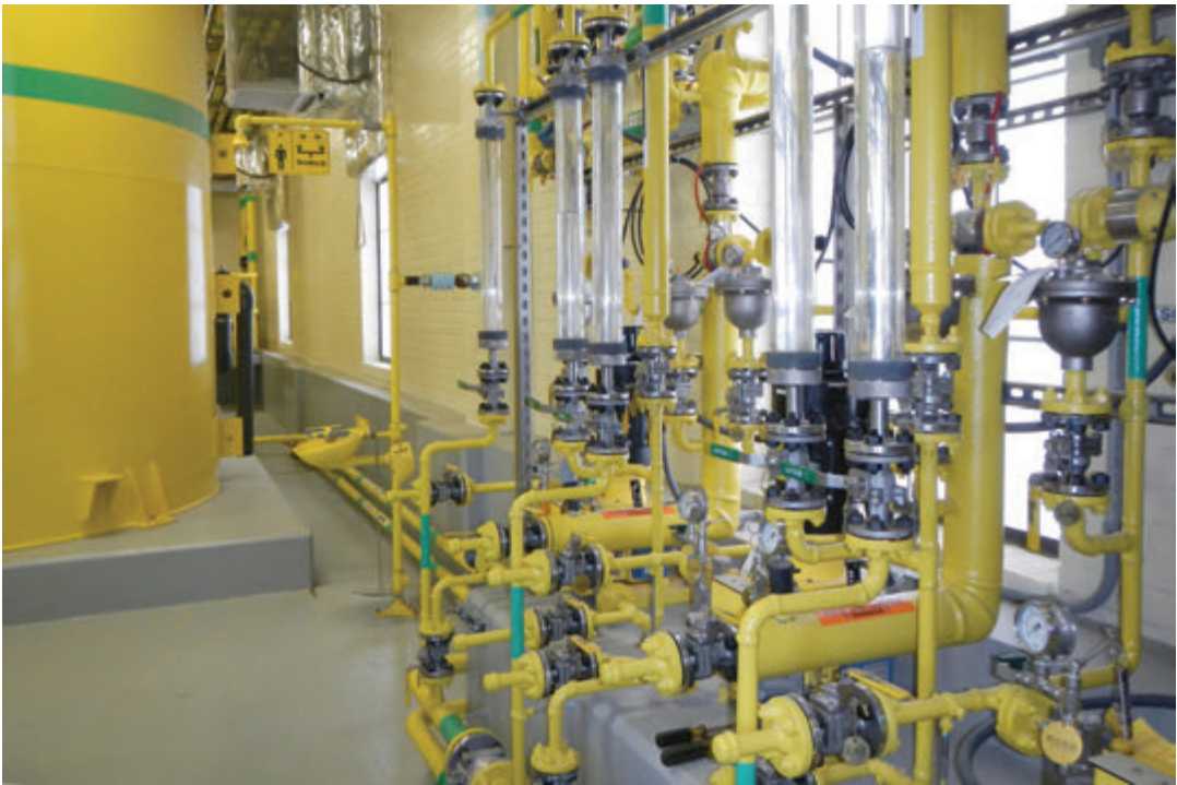
Recent Construction - Sodium Hydroxide System
