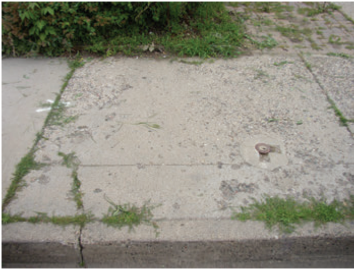
Deteriorated Sidewalk
