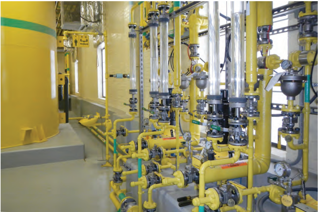
Recent Construction - Sodium Hydroxide System
