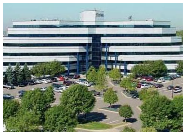
Figure 31. Broadway Place West, winner of the Building Energy Performance Award for lowest energy use intensity (42 kbtu/ft/yr) for the business category
