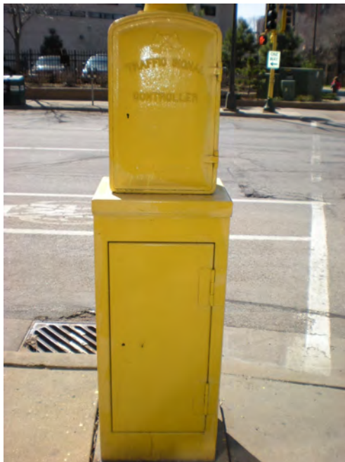
Obsolete Signal Controller and Cabinet
