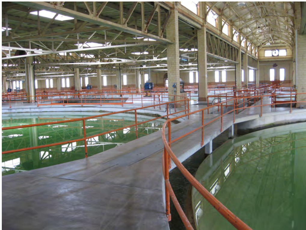
Interior Process of Softening Plant
