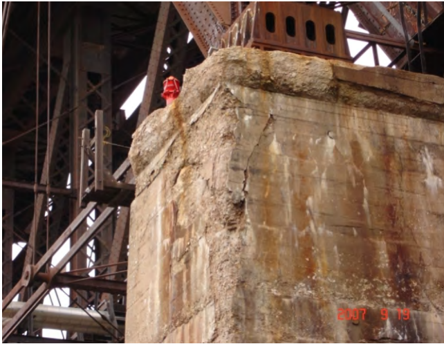
Pier Cap Deterioration Bridge #9 Ped/Bike Bridge over Mississippi River
