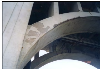
Arch Deterioration
