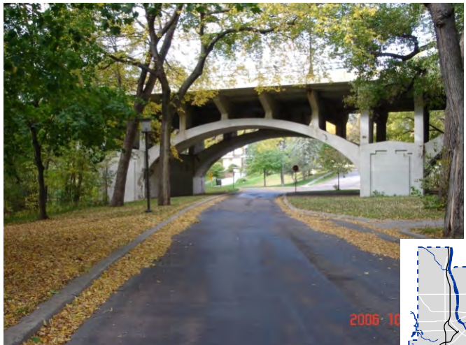
10th Ave SE Bridge over Mississippi River - New Bicycle Railings to Meet Current Standards
