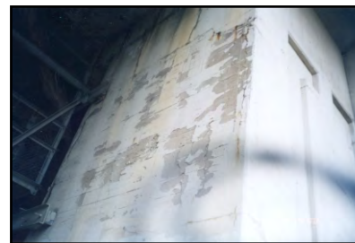
Pier Deterioration
