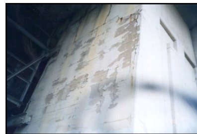
Pier Deterioration
