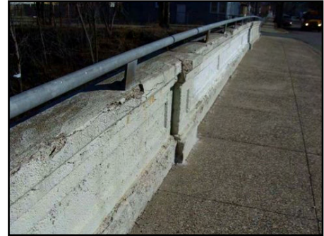
Railing Deterioration
