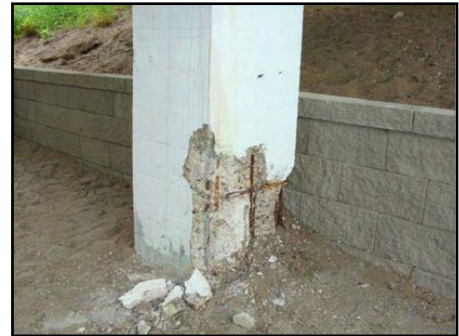
Pier Column Spalls
