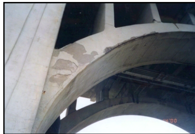
Arch Deterioration
