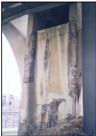
Pier Deterioration
