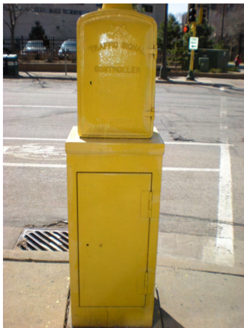
Obsolete Signal Controller and Cabinet
