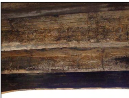
T-Beam Stem Deterioration
