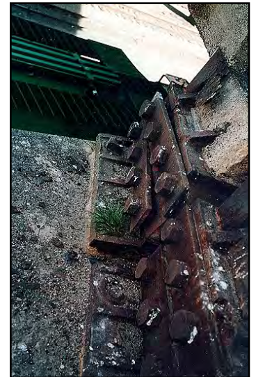
Bearing Corrosion
