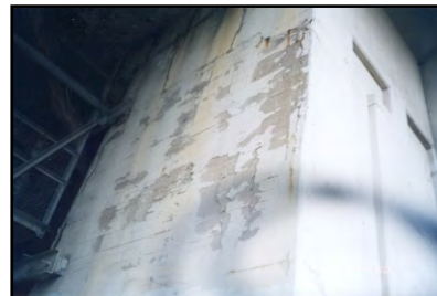
Pier Deterioration
