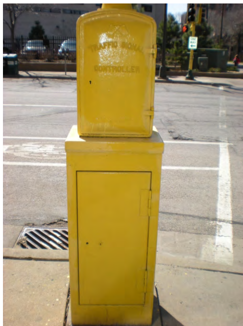
Obsolete Signal Controller and Cabinet
