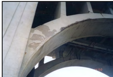
Arch Deterioration
