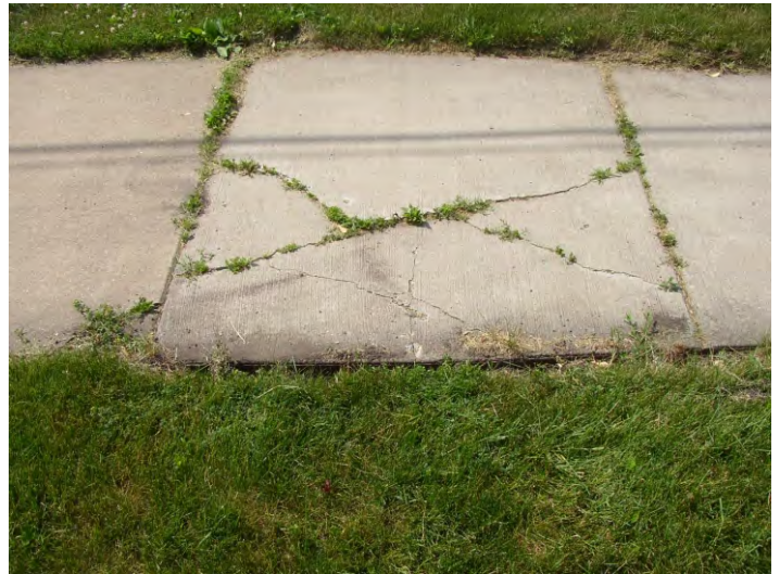
Broken Sidewalk
