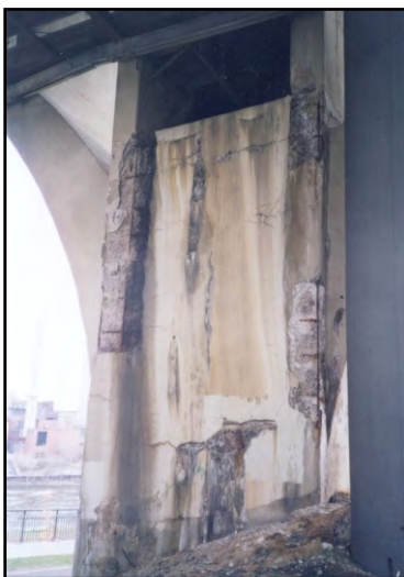
Pier Deterioration
