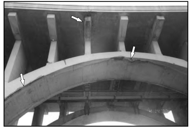
Arch and Floor Beam Deterioration
