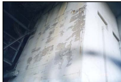
Pier Deterioration
