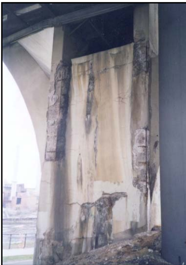
Pier Deterioration
