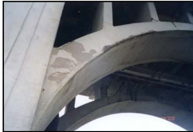
Arch Deterioration
