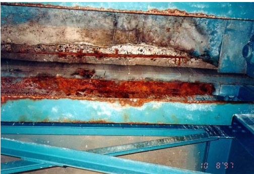
Corroded Deterioration
