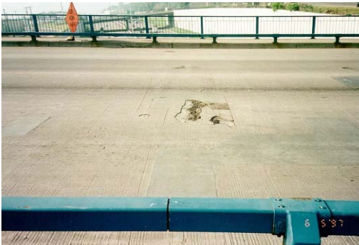
Deck Deterioration
