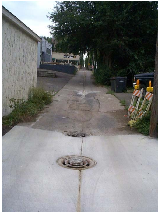
Completed Storm Drain Project
