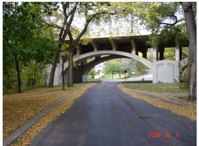
Nicollet Ave Bridge
