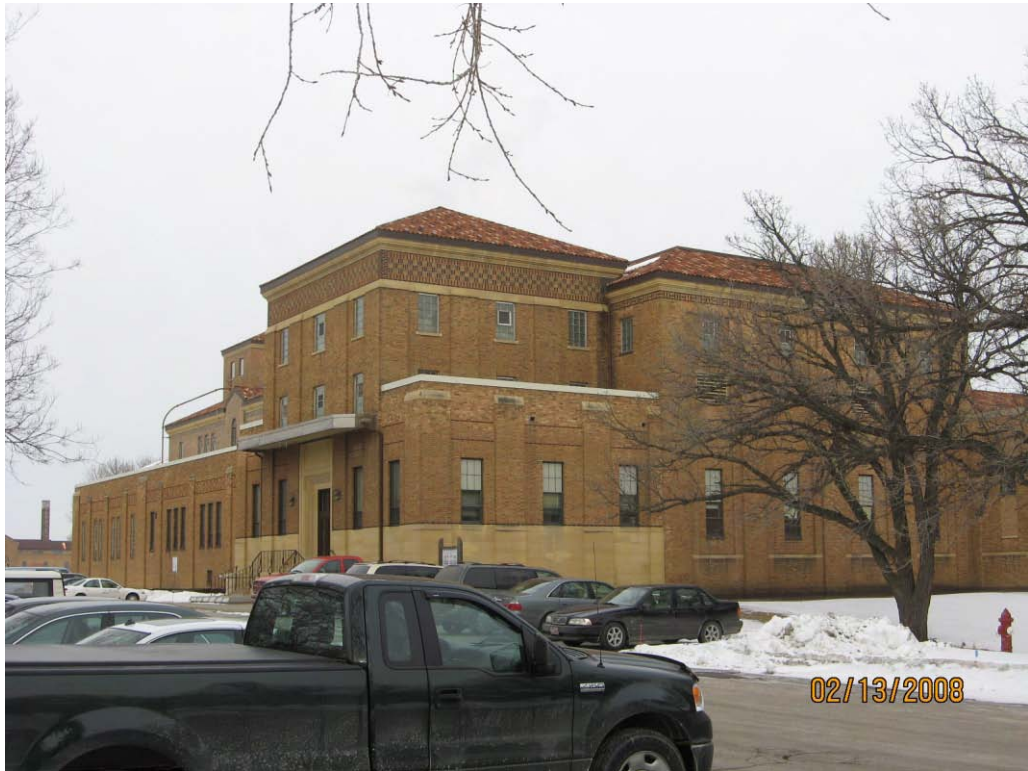
Fridley Softening Plant, completed around 1940
