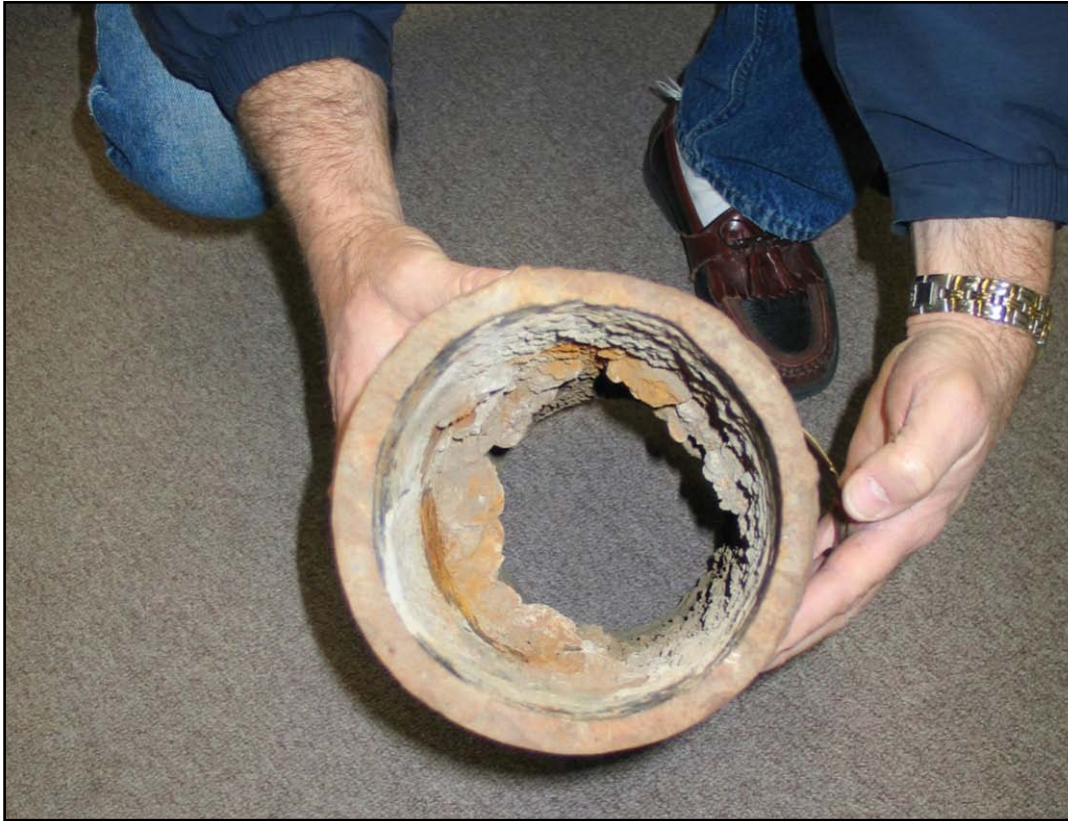
Water pipe before cleaning
