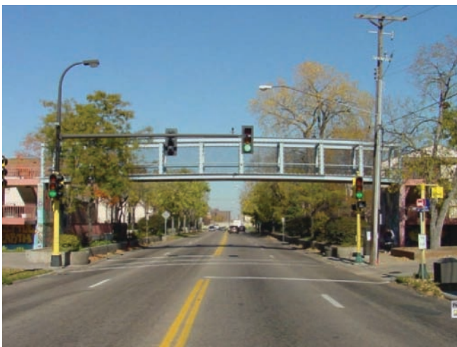
Pedestrian Bridge Painting Project to cover Lead Based Paint
