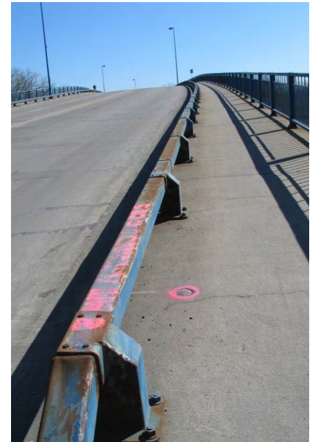
Corroded Railing
