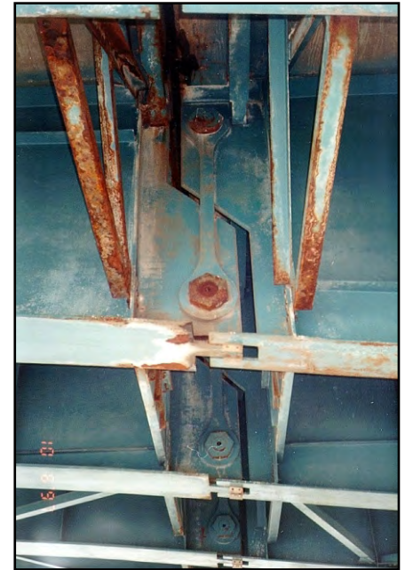
Corroded Pin Hinge & Bracing
