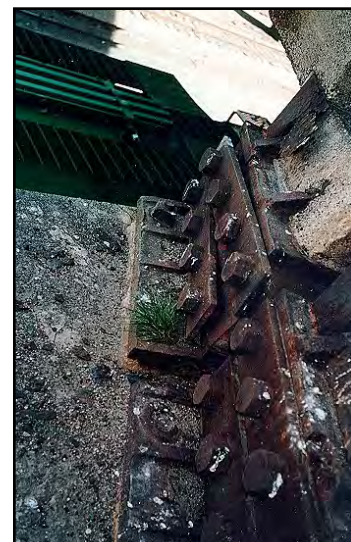
Bearing Corrosion
