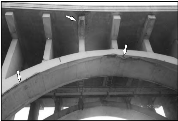
Arch and Floor Beam Deterioration
