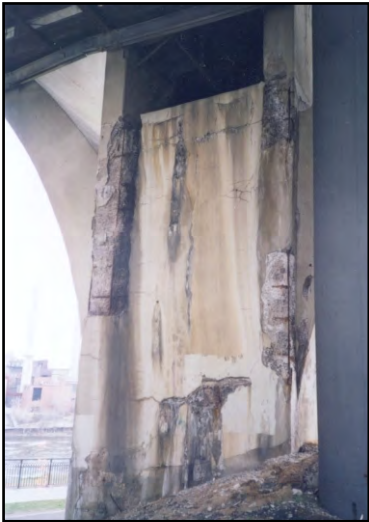
Pier Deterioration
