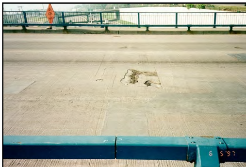
Deck Deterioration
