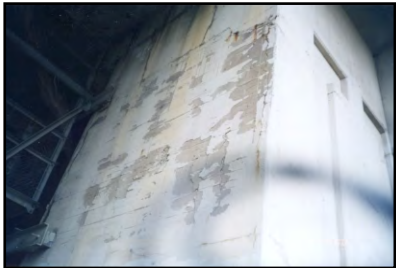
Pier Deterioration
