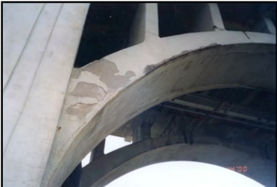
Arch Deterioration
