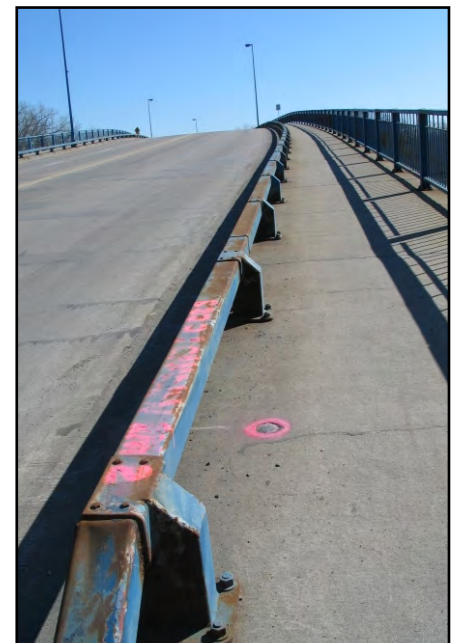
Corroded Railing
