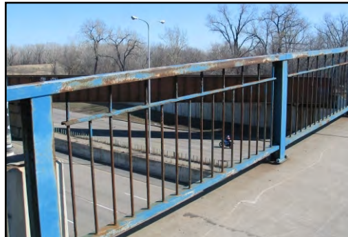
Corroded Guard Rail
