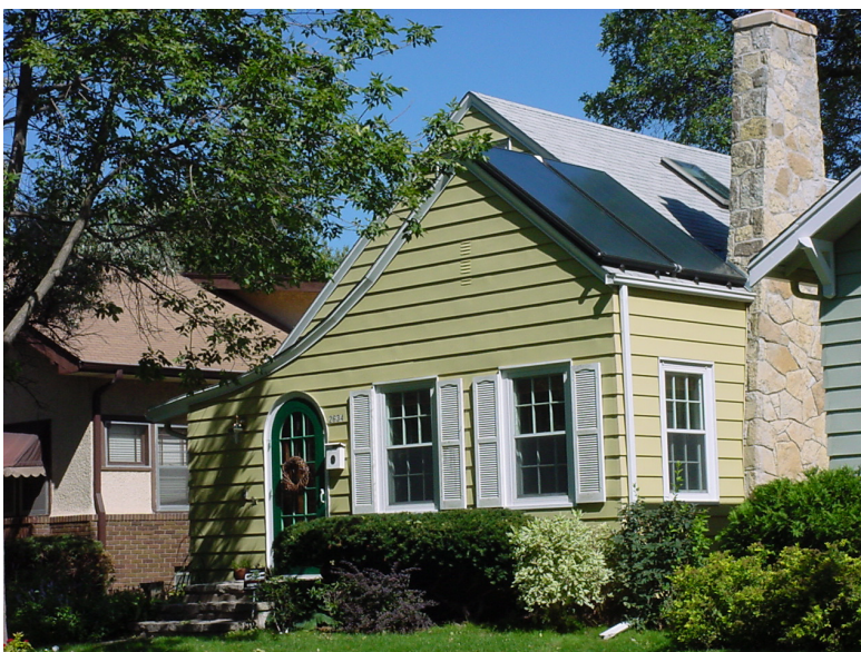
This north Minneapolis home has both a solar photovoltaic (electrical) and a solar thermal (hot water) system that meets about 25 percent of its residents' energy needs.
