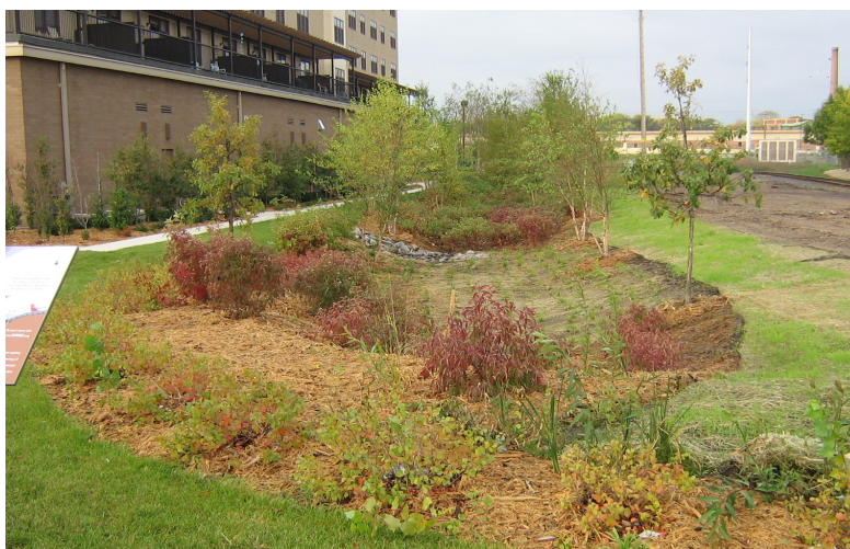
This new development has two rain gardens – one for rooftop runoff and the other for the parking lot. New rain gardens reduce the rate and amount of runoff, improve water quality, promote stormwater awareness, and add habitat and visual interest.
