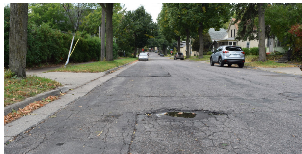
This intersection shows a "poor" asphalt pavement condition
