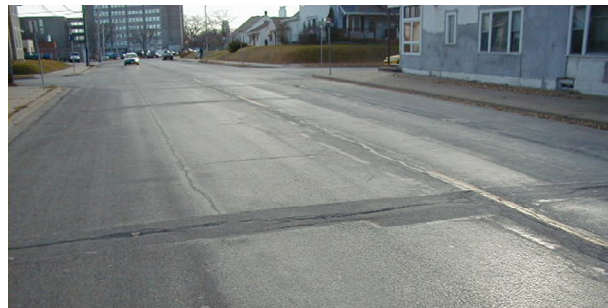
This street would be considered a "fair" asphalt pavement condition
