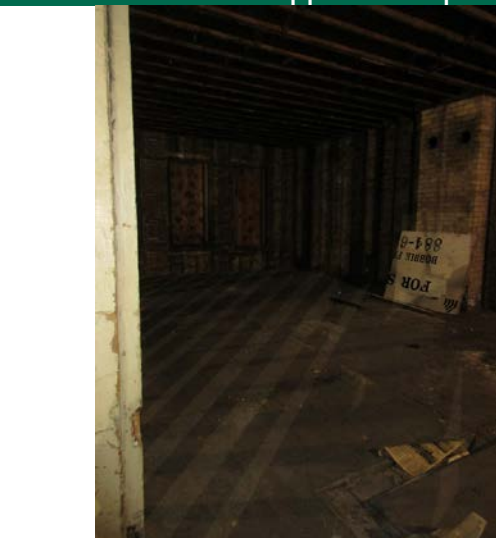
View of inhabitable upper floor space
