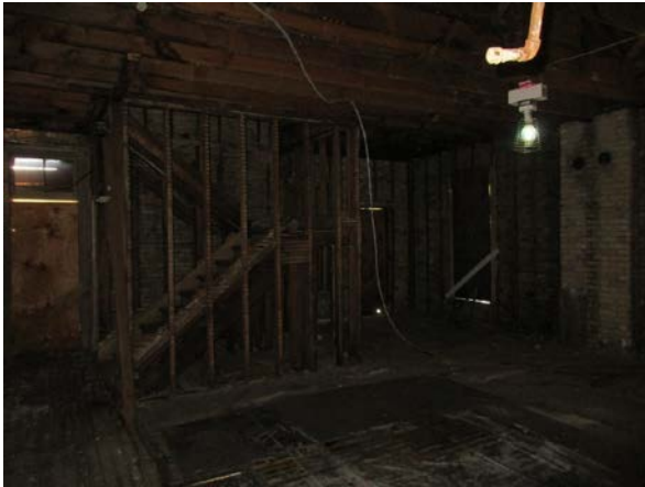
View of inhabitable upper floor space
