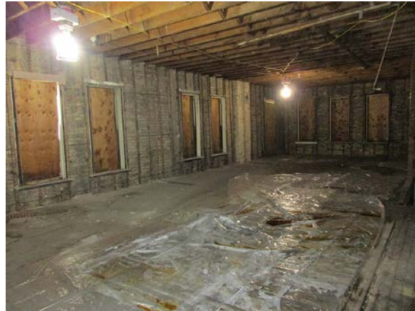
View of inhabitable upper floor space
