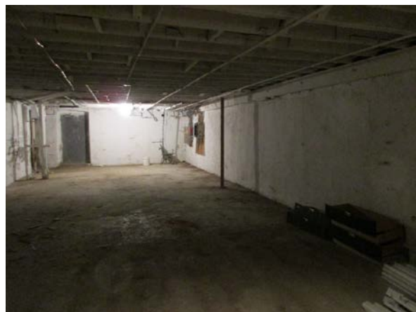
View of inhabitable basement space
