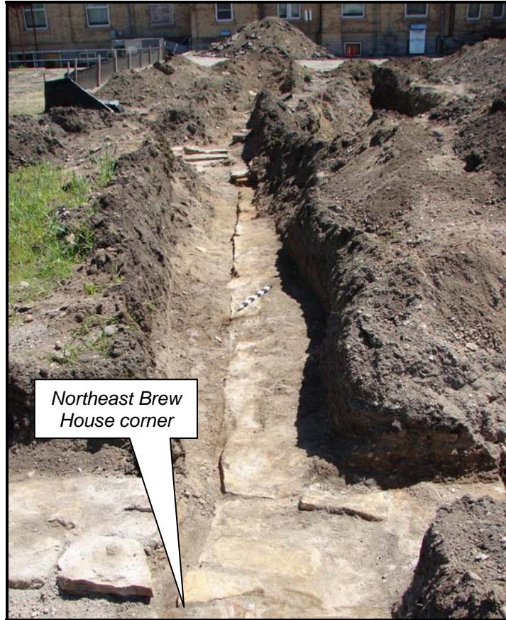
FIGURE 23. NORTHEAST CORNER AND EXPOSED SECTION OF EAST WALL OF THE ORTH BREW HOUSE, VIEW TO SOUTHEAST
