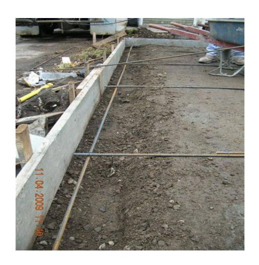
• ½" anchor bolts shall extend 7" min. into masonry or concrete and spaced a maximum of 6' on center and within 12" from each end. **MNSBC** 403.1.6
