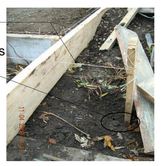
Inspector approves **Thickened** perimeter slab base preparation before concrete is poured.
