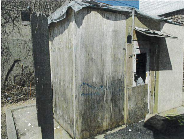
Treated Plywood Shed – Southeast Corner of Shed
