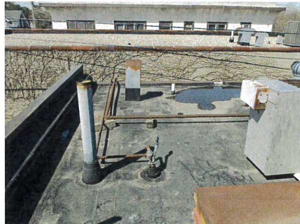
2" x 2" Treated Wood Blocks - Roof
