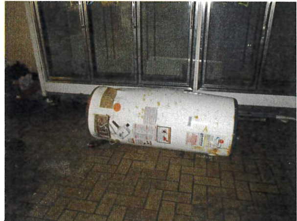
Water Heater and Freezer – Convenience Store
