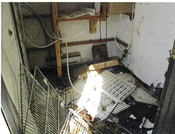
Municipal Solid Waste – Janitor's Closet
