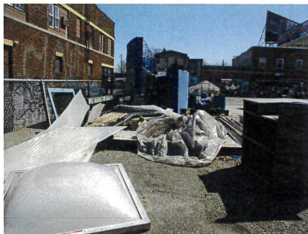
Treated Plywood and Plywood Garden Structure – North Side of Site
