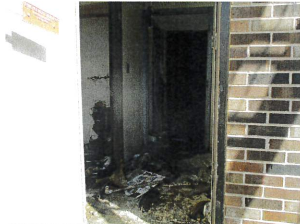
Municipal Solid Waste - South Entrance to Building
