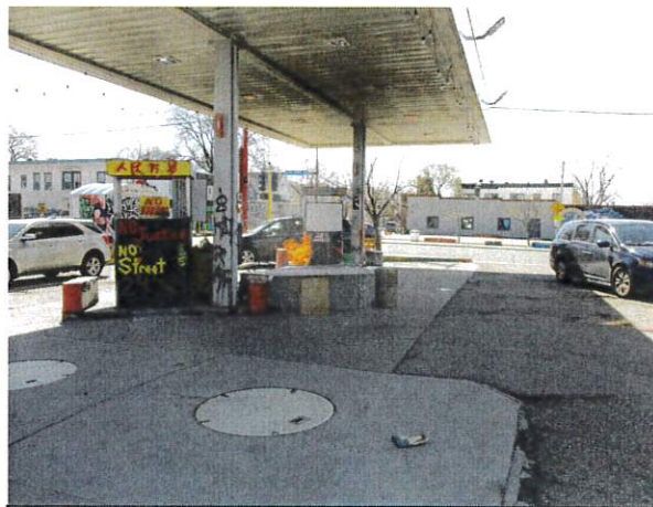
Underground Storage Tanks – Northeast Area of the Site, Fuel Pumps East Side of the Site
