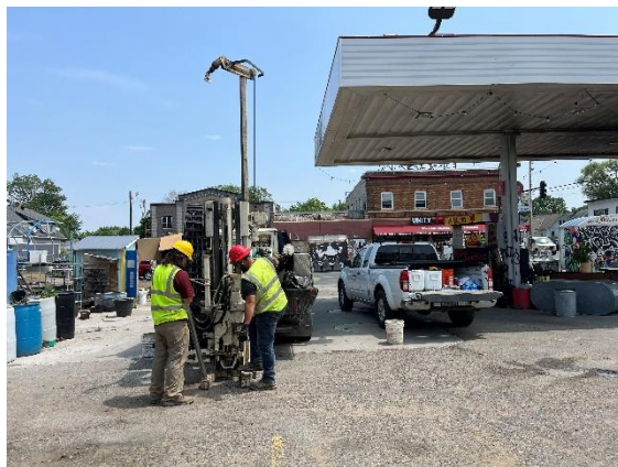
SB-3, View to the East
