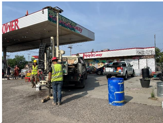
SB-1, View to the West Southwest
