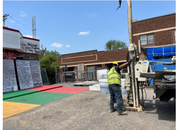
SB-4, View to the North Northwest
