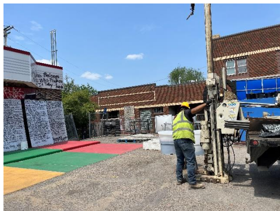
SB-3, View to the North Northwest
