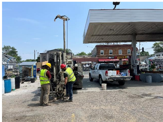
SB-2, View to the South
