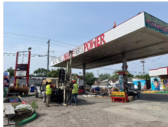
SB-2, View to the southwest
