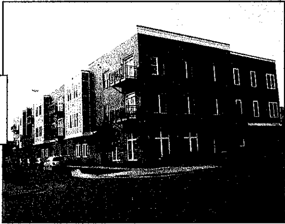
Northwest corner Cedar Avenue and 29 th Street
