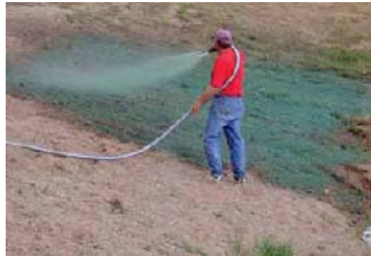
Hydrodraulic soil stabilizers promote the rapid growth of vegetation and prevent erosion.
