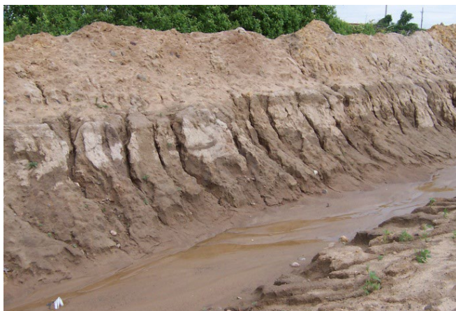
Subsoil erosion at a construction site.
