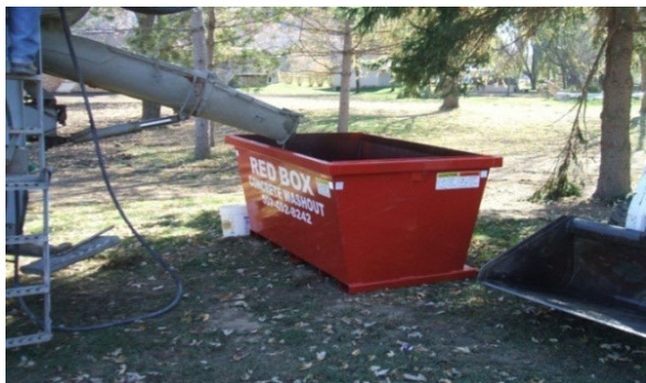
Concrete washout service
