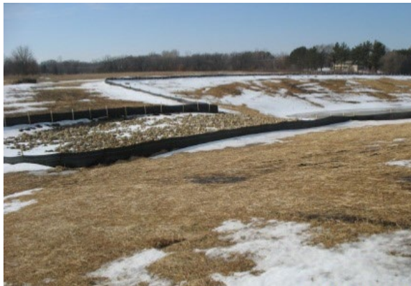
Silt fence used as perimeter control
