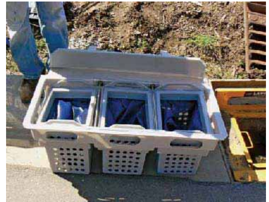
Stormwater inlet protection BMPs can be inserted into a catch basin to trap sediment from a construction site before it enters a storm sewer.
