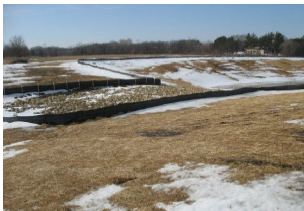
Silt fence used as perimeter control
