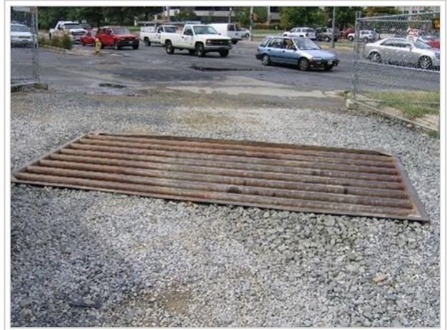
Example shaker rack installation. Source: Tetra Tech.
