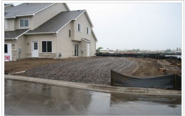
Properly constructed BMP for vehicle tracking.
