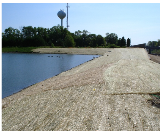
Erosion control blanket stabilizes pond slopes.
