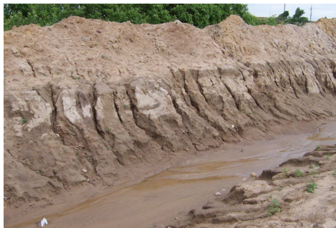
Subsoil erosion at a construction site.
