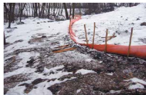
Regular maintenance is needed to ensure that a site's perimeter control is functioning properly.
