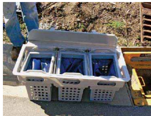
Stormwater inlet protection BMPs can be inserted into a catch basin to trap sediment from a construction site before it enters a storm sewer.
