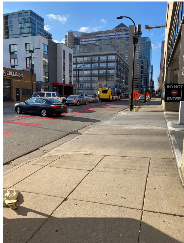
Figure 6 – Traffic Exiting Purple Ramp to 7 th St. and Temporary Lane Closure Beyond
