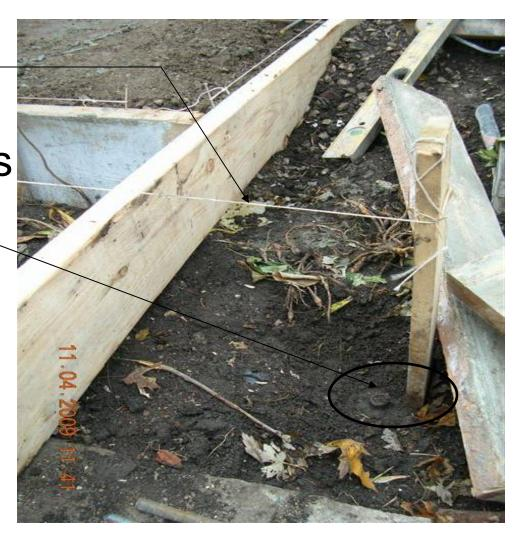
Inspector approves **Thickened** perimeter slab base preparation before concrete is poured.
