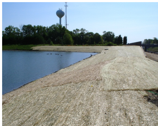
Erosion control blanket stabilizes pond slopes.
