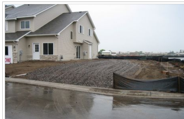
Properly constructed BMP for vehicle tracking.
