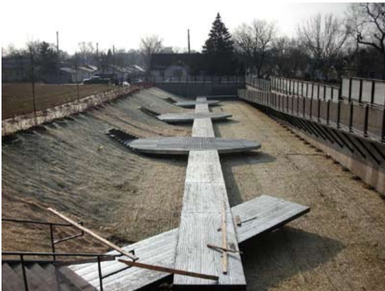
Folwell School Interpretive Rain Gardens (under construction) This project removed nearly two acres of asphalt and boosted the school’s environmental curriculum. Students will use the rain garden walkway to learn about managing stormwater.
